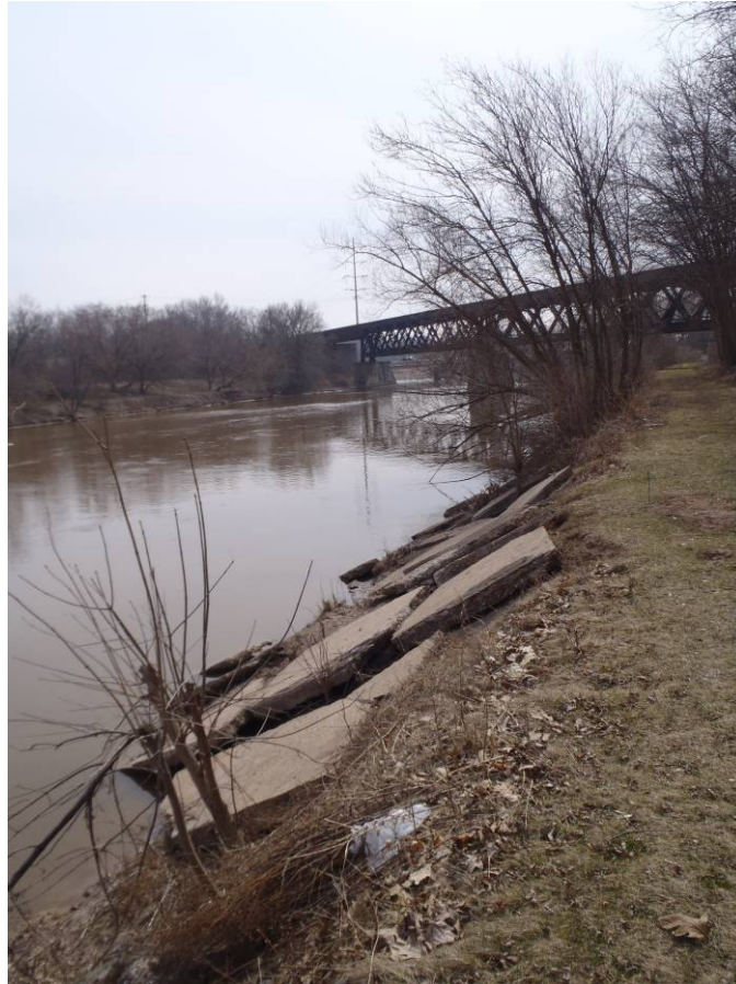
Photo 5: Concrete Slab and Asphalt Rip-Rap.
