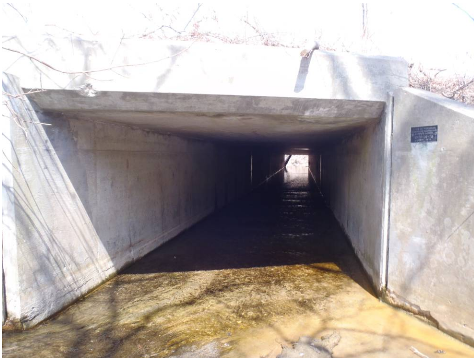
Photo 12: The upstream end of the culvert under Indiana Avenue.
