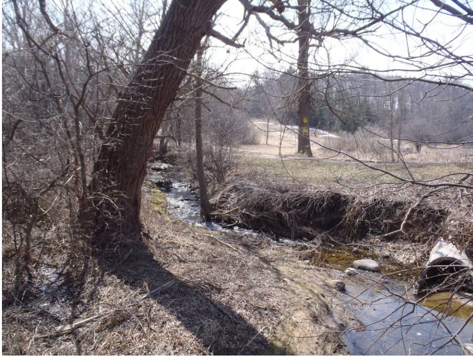
Photo 11: The tributary stream and culvert connecting to the southeast wetland.
