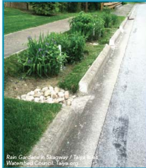
Infiltration basins behind curb cuts
