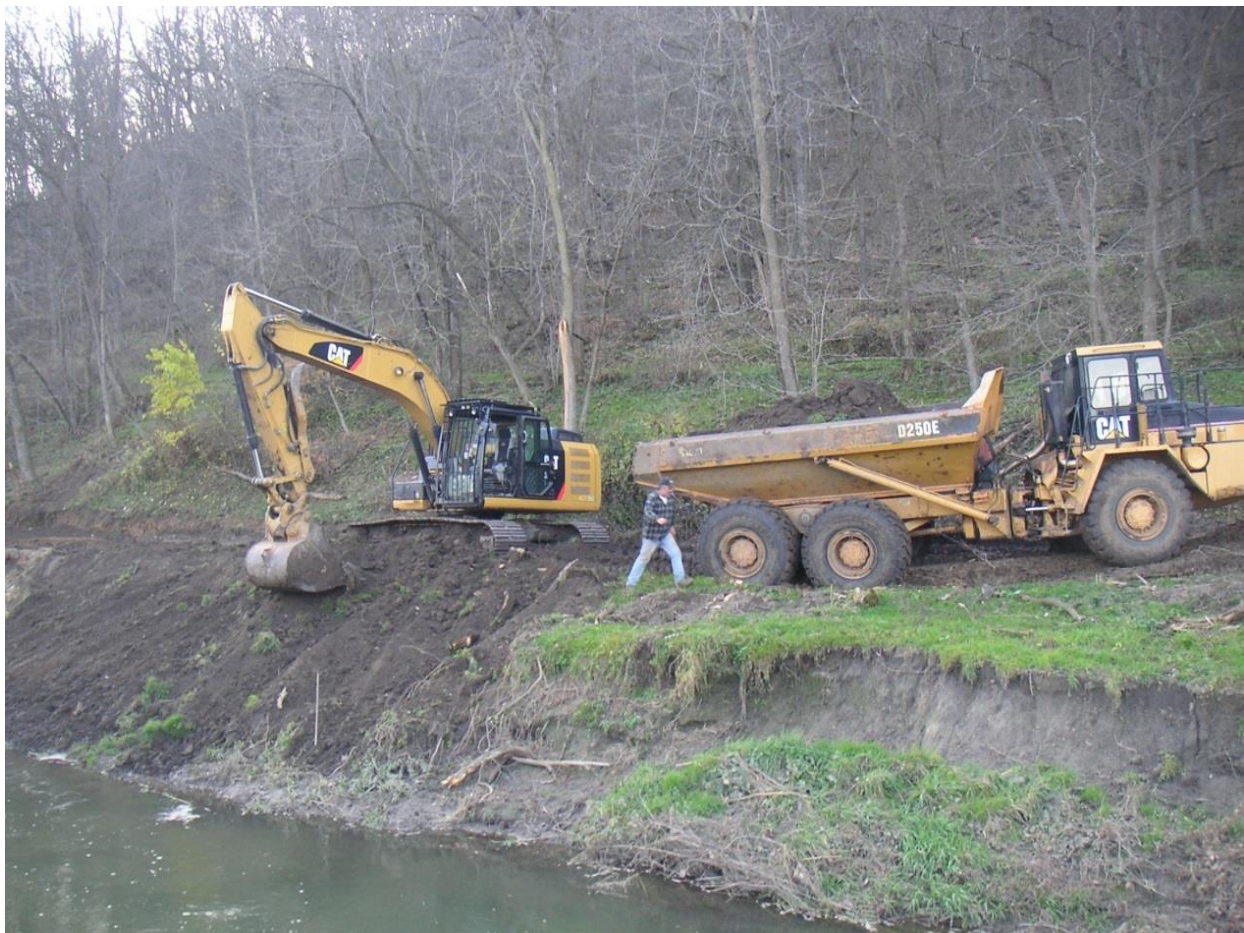
A section of stream against the hillside being tapered. Notice the large section of bank that sluffed off during one of the large rain events that occurred while the work was in progress. This happened in several other areas as well.
