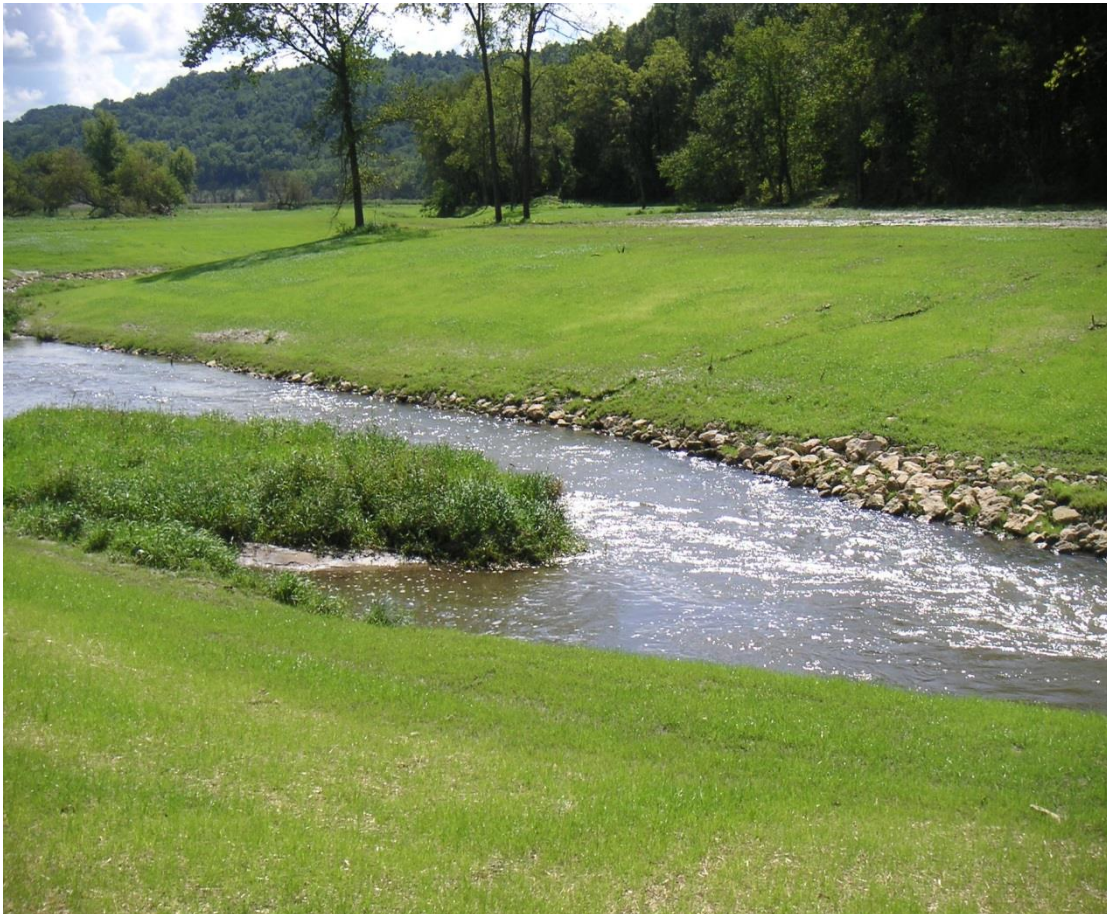
A back water area created when a tall vertical bank was tapered to an island
