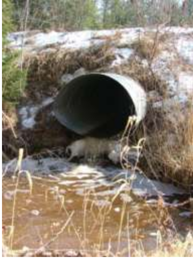
Figure 2.25. Example of a typical perched culvert in the Marengo River Watershed.
