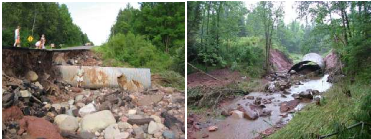
Figure 2.27. Examples of failed culverts in the Marengo River Watershed.
