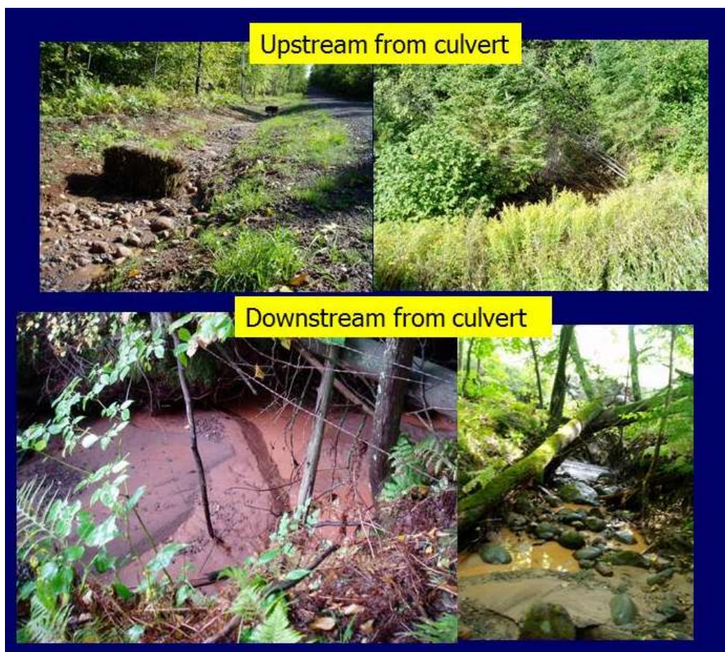
Figure 2.26. Examples of typical road/stream interaction at culverts in the soil transition zone of the Marengo River Watershed (courtesy of F. Fitzpatrick). Sediment accumulation upstream and erosion downstream.
