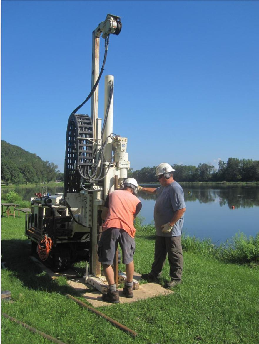
FIGURE 3.5 - GEOPROBE DRILLING: JIM RAUMAN AND JASON SMITH OF THE U.S. GEOLOGICAL SURVEY INSTALLING A GROUNDWATER MONITORING WELL NEAR LAKE MARION.
