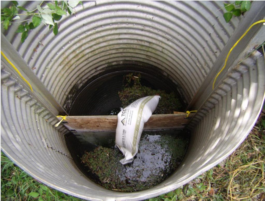
FIGURE A7.1 - PHOTO OF BOARDS BLOCKING A CULVERT.
