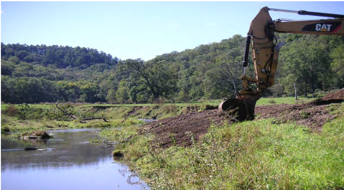
Starting to shape the high banks and help the stream reconnect to the floodplain
