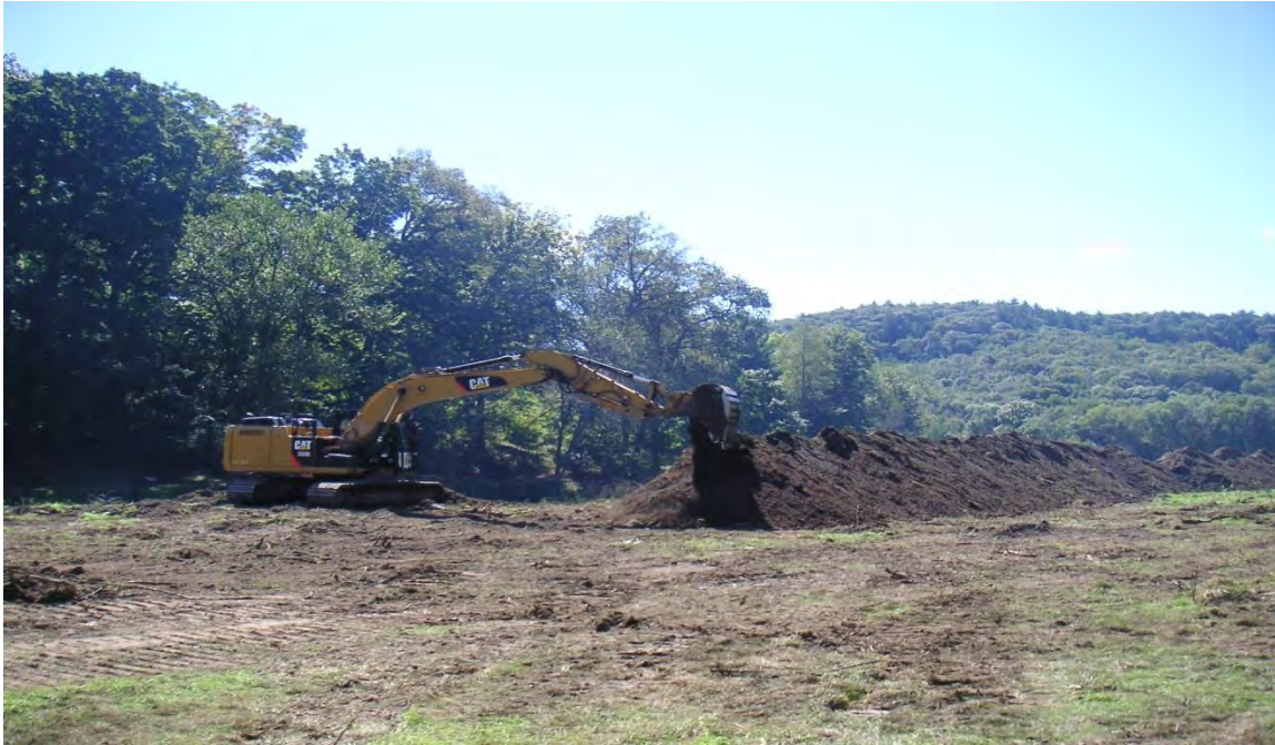
A large amount of bank spoil was removed from the immediate flood plain
