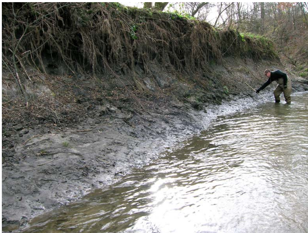
Figure E-6. Typical bank erosion along Little Willow Creek downstream of Spiral Road
