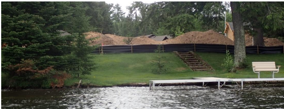
Figure 9. There was some major construction adjacent to Little Crooked Lake in 2020. Silt fences appeared to be properly placed.
