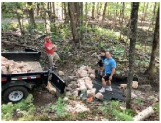
ground fabric was laid over the swale and tucked into the upstream side of the bed. It was then covered with quarry rock weighing between 20-70 pounds, puzzled in with smaller rock to hold it all together under the force of rushing water.
