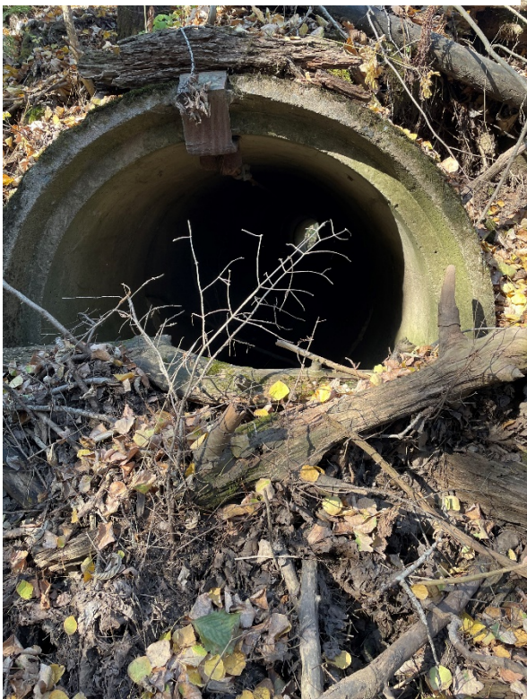
Photo 6. (Left) Upstream end of Neuman Road culvert. Large debris barrier was present.
