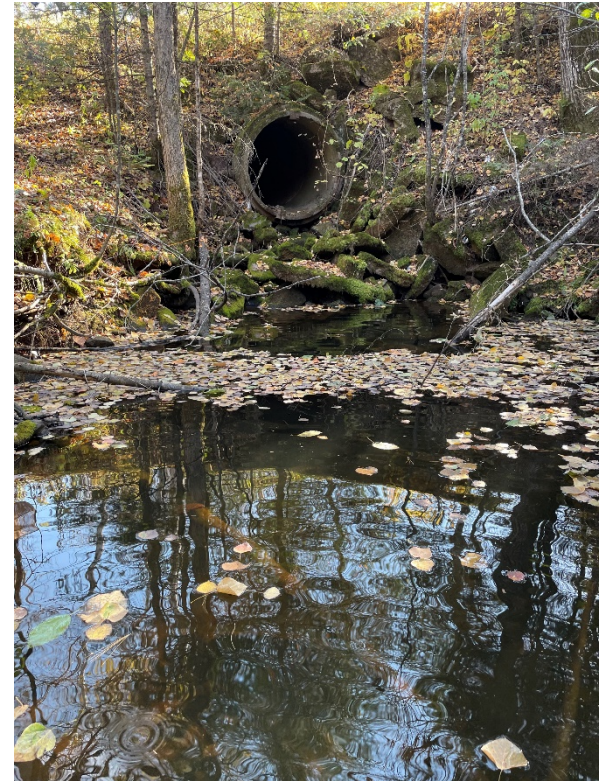
Photo 8. (Right) Downstream end of Neuman Road culvert. Rock pile at the mouth of the culvert is about 1m high.
