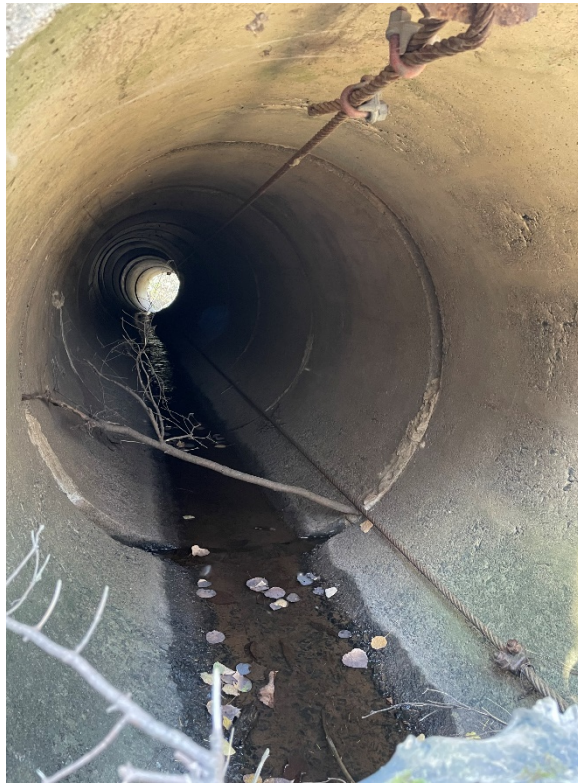
Photo 7. (Center) Inside of Neuman Road culvert viewed from the upstream end. There is a rise and bend in the culvert.
