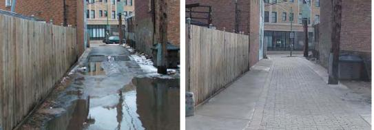
Figure 17. Alley with impervious pavement and poor drainage (left); alley with pervious pavement resulting in no standing water (right).
