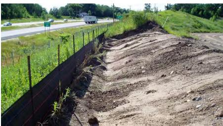
Figure 27. Installed silt fence will minimize sediment from leaving a site and entering surface waters.
