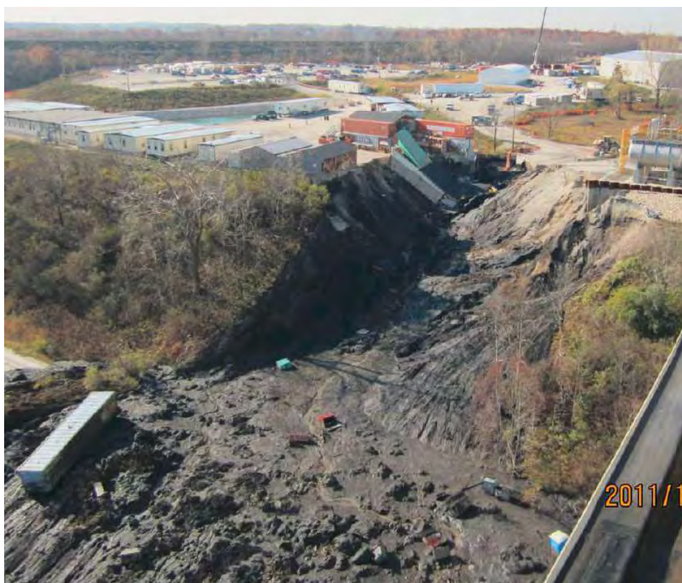
October, 2011 bluff failure at We Energies Oak Creek Power Plant. Source: WDNR & We Energies
