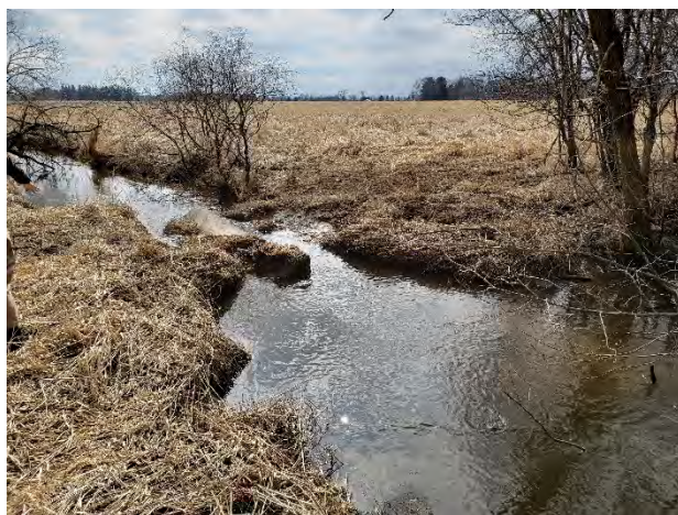
Photo 2. Mason Creek - Upper culvert f/ds (~ Sta. 10+00)
