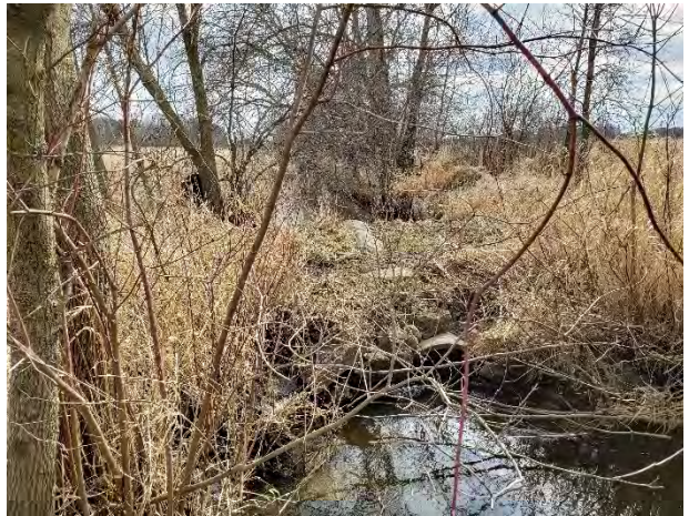
Photo 6. Mason Creek – Lower Culvert f/ds (~ Sta. 15+00)
