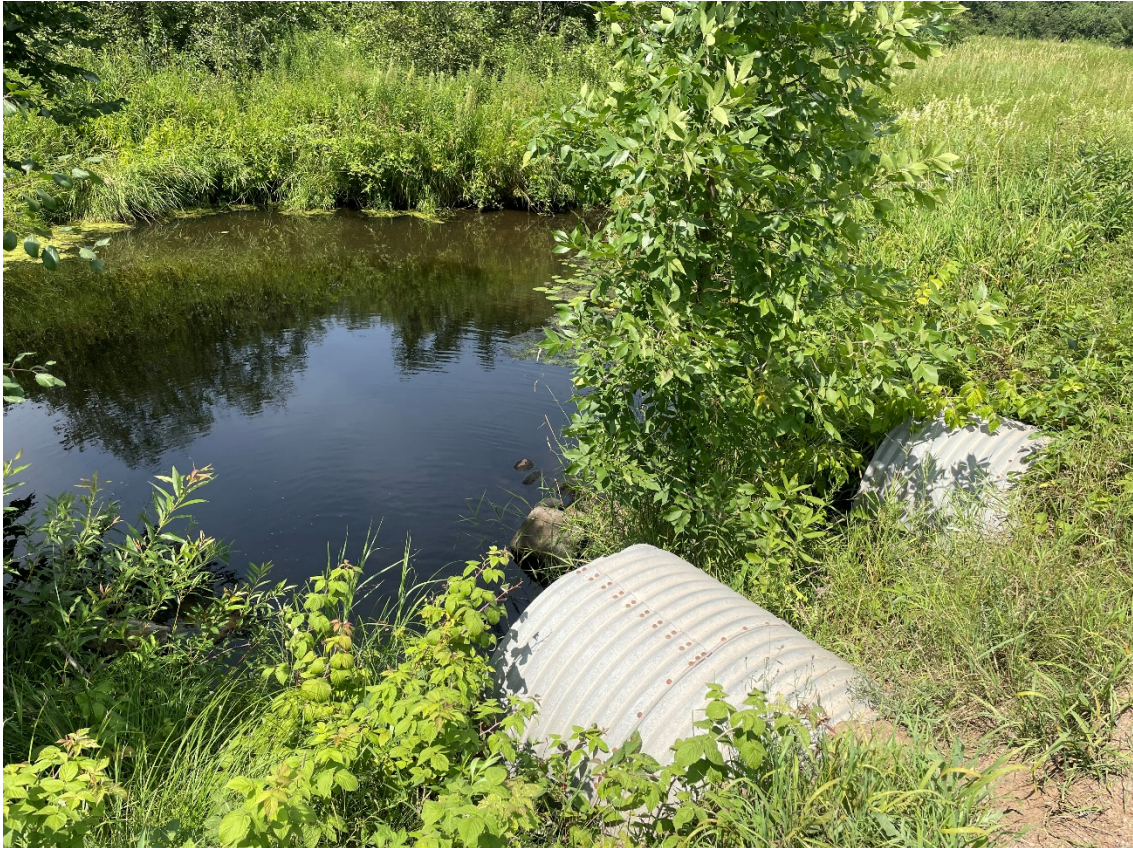
Photo 10. S. Branch of Beaver Brook looking downstream at 25 th Street.
