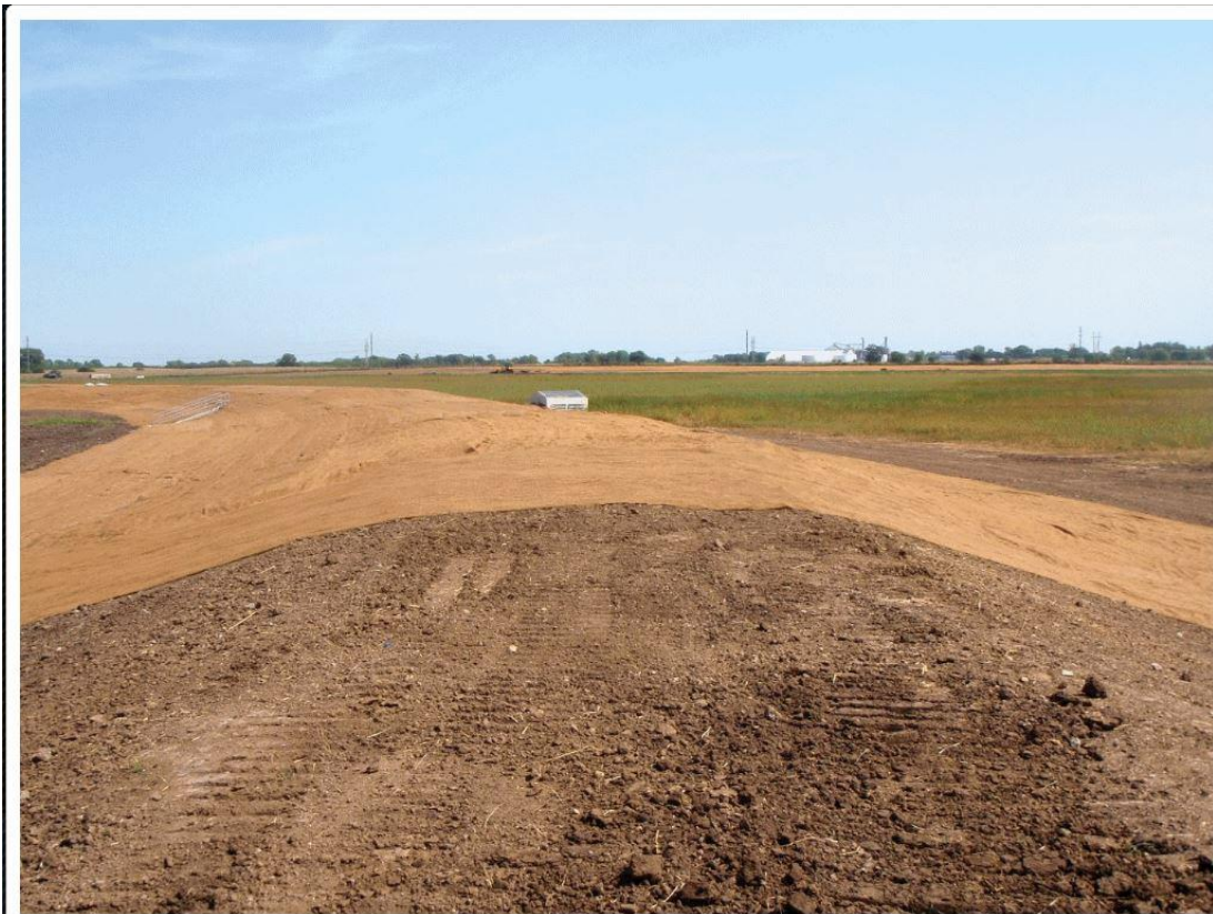
Photo 2: James Road Detention Basin Outlet Under Construction. Photo courtesy of City of Oshkosh Public Works Department 2013.
