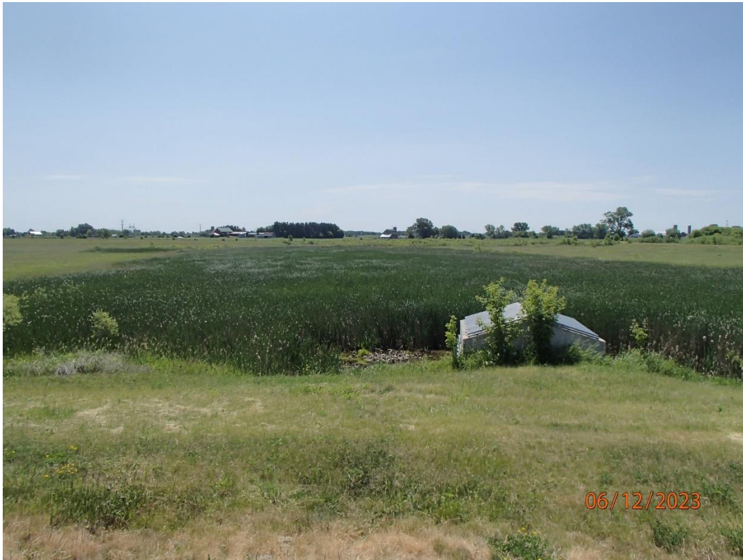
Photo 5: James Road Retention Basin at time of June 12 th , 2023, monitoring event. Photo taken by D. Bolha.
