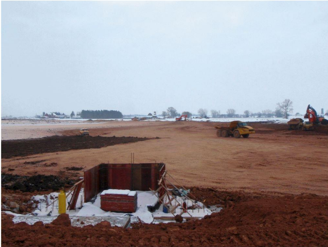
Photo 1: James Road Detention Basin Under Construction. Photo courtesy of City of Oshkosh Public Works Department 2013.
