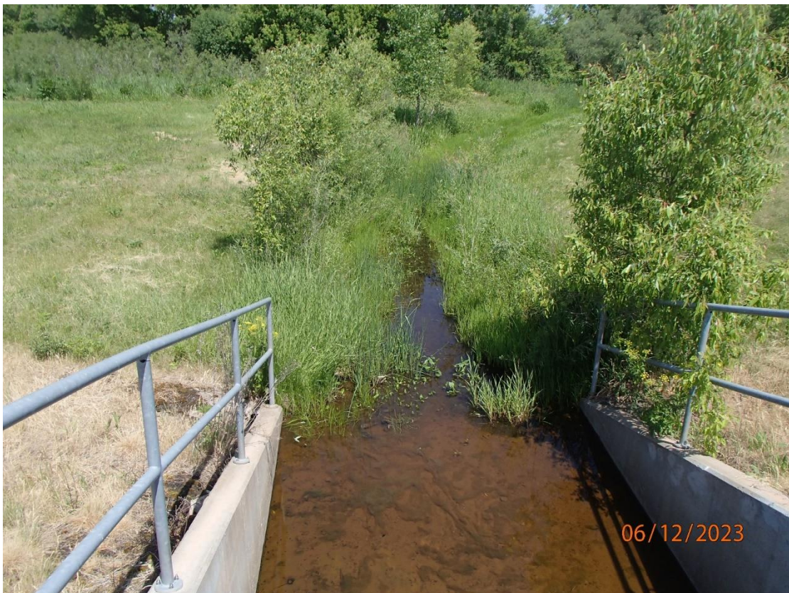
Photo 6: James Road Retention Basin Outlet at time of June 12 th , 2023, monitoring event. Photo taken by D. Bolha.
