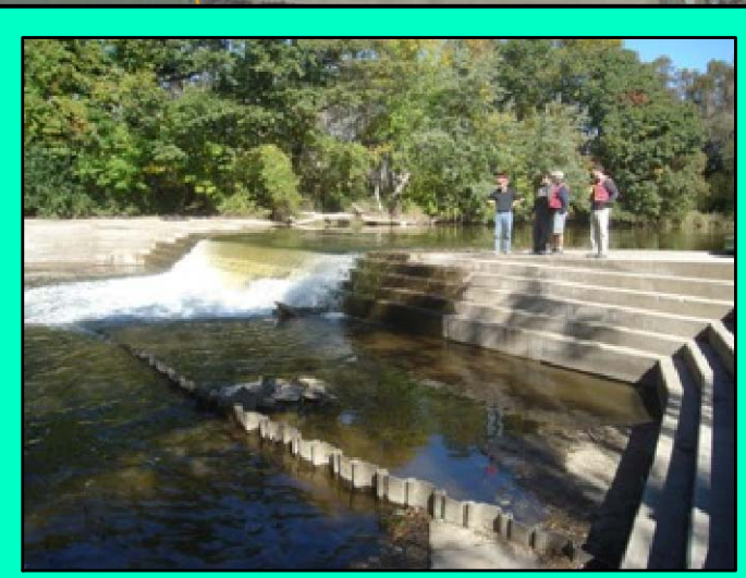
Aquatic Issues - Walderhaus Dam
