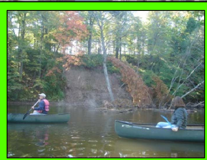
Bank Stabilization - River Bank Slough
