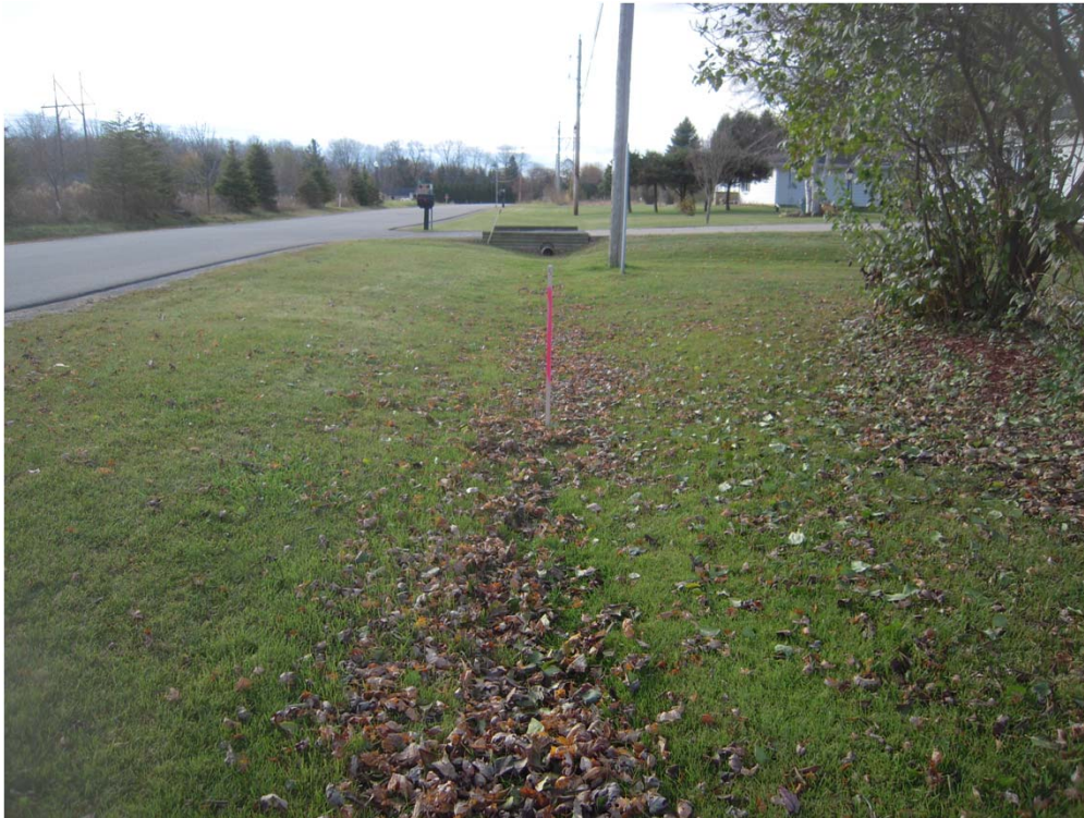
Photo 5. Viewing south at Sample Point 5
