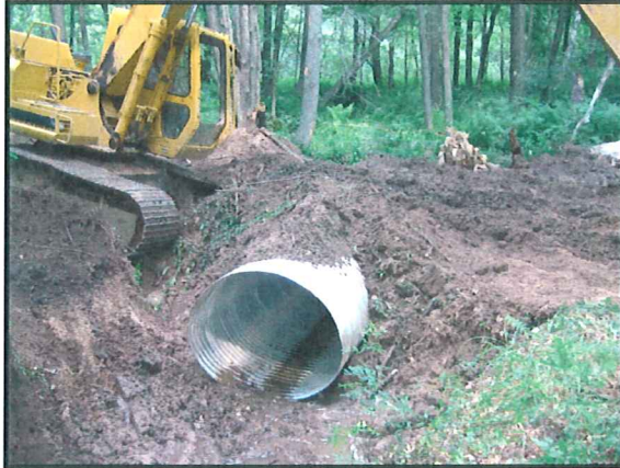
Figure 1. Paint Creek Riparian Buffers - Brian Phillips Stream Crossing Construction
