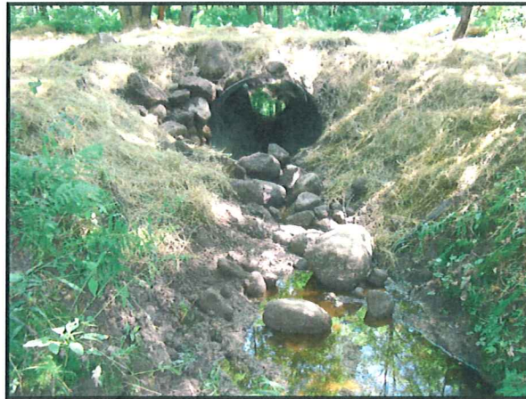
Figure 2. Paint Creek Riparian Buffers - Brian Phillips Stream Crossing Construction
