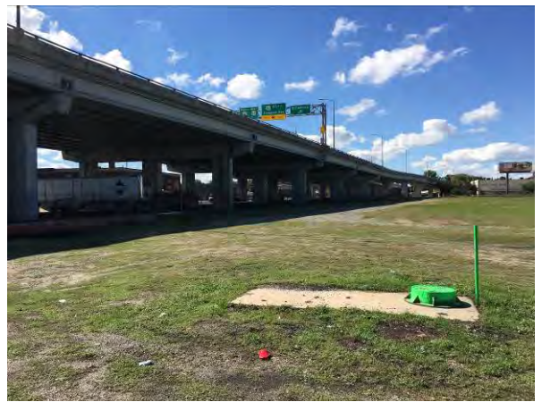
Photo #10 Man-hole access point on the southeast corner of the Parcel – looking west
