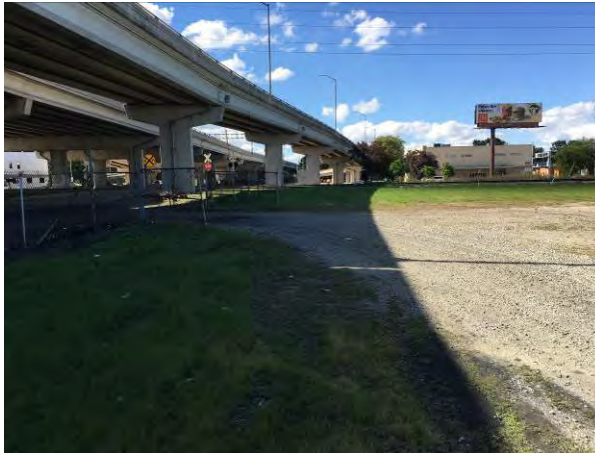
Photo #13 Open gate accessing the Parcel
