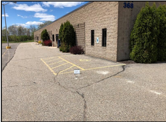
Hydraulic Push Soil Boring G7.
