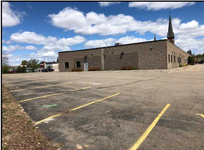
View northeast toward on-site structure.
