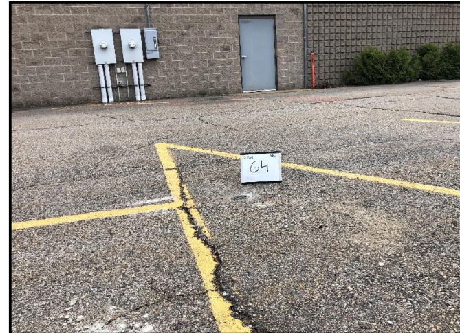
Hydraulic Push Soil Boring G4.
