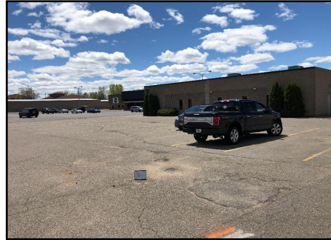
Hydraulic Push Soil Boring G11.
