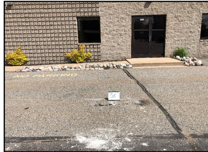
Hydraulic Push Soil Boring G6.
