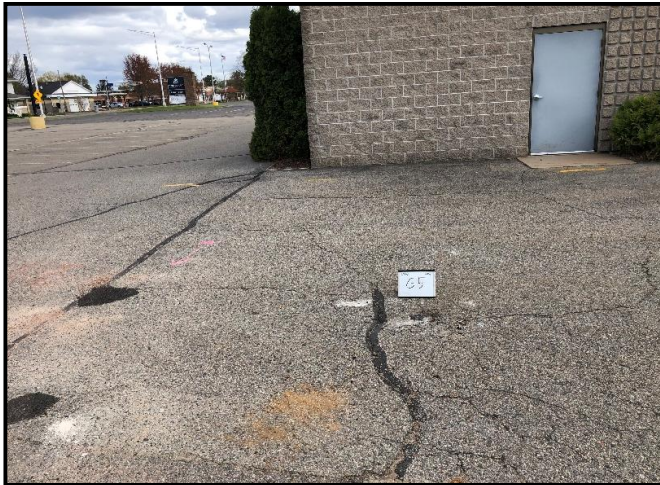
Hydraulic Push Soil Boring G5.
