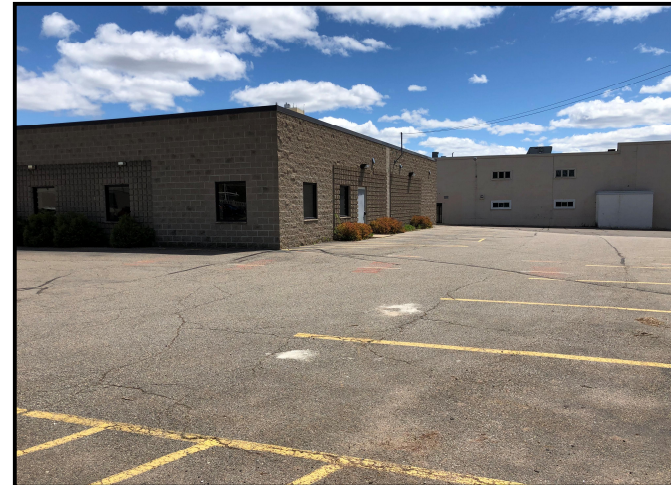
View southeast toward on-site structure.
