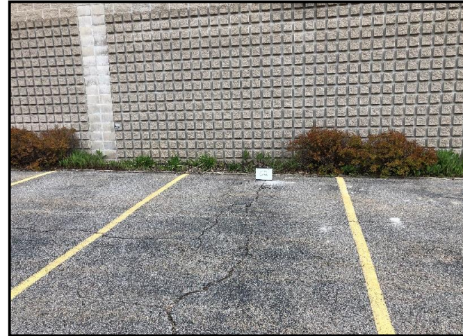
Hydraulic Push Soil Boring G2.
