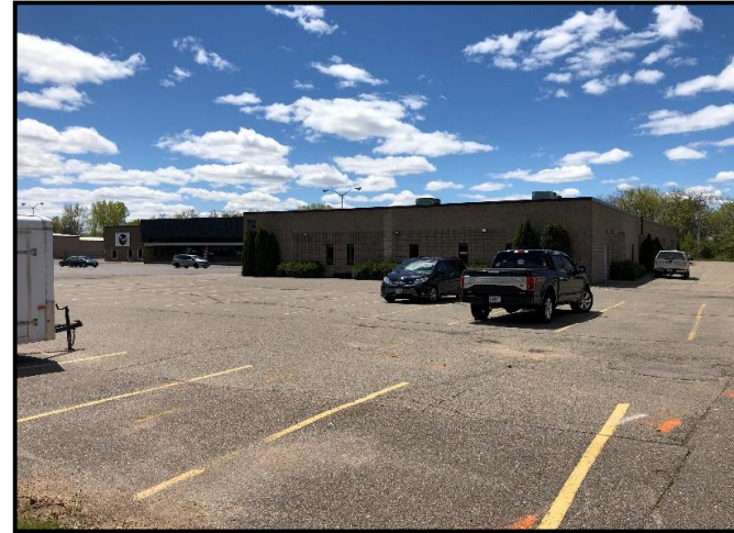
View southwest toward on-site structure.
