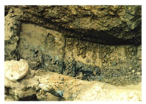
Description Soil staining of 2,000 gallon kerosene UST
