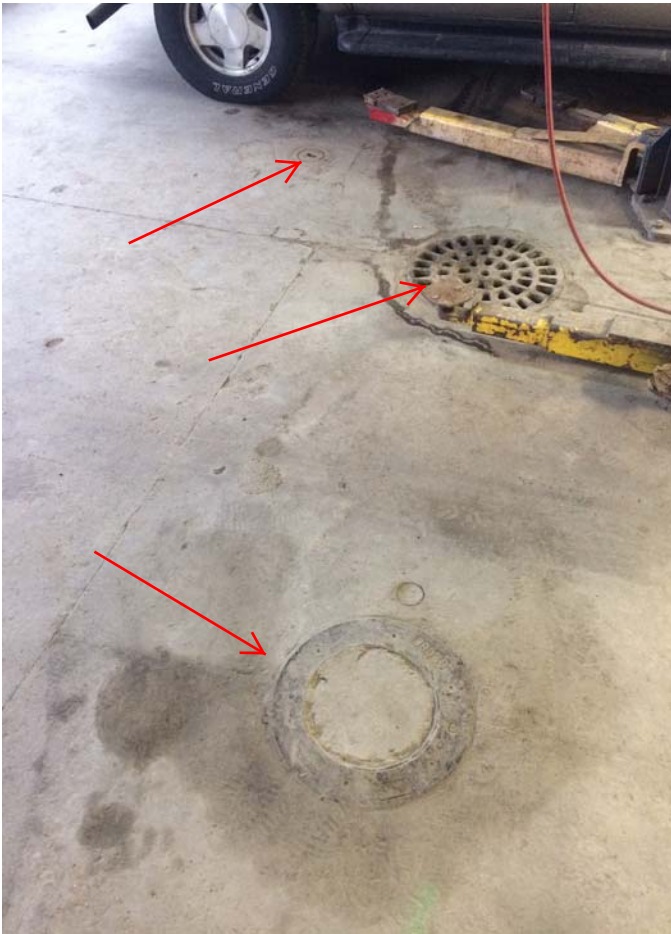
#5 - View of fmr. lift, catch basin, and MW-1
