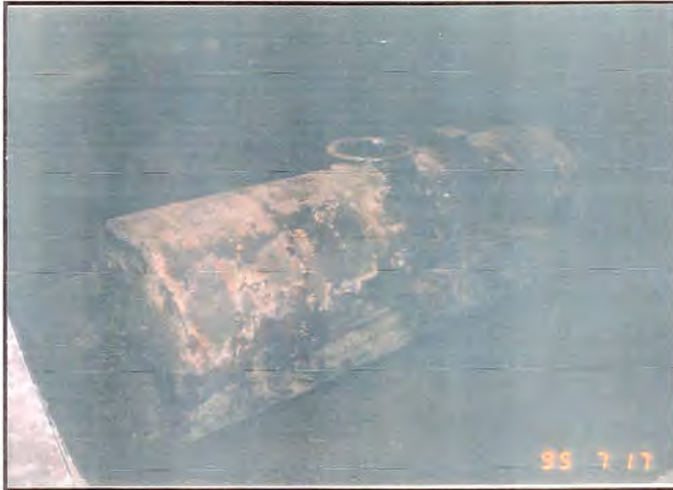
Tank 9 inside excavation.
