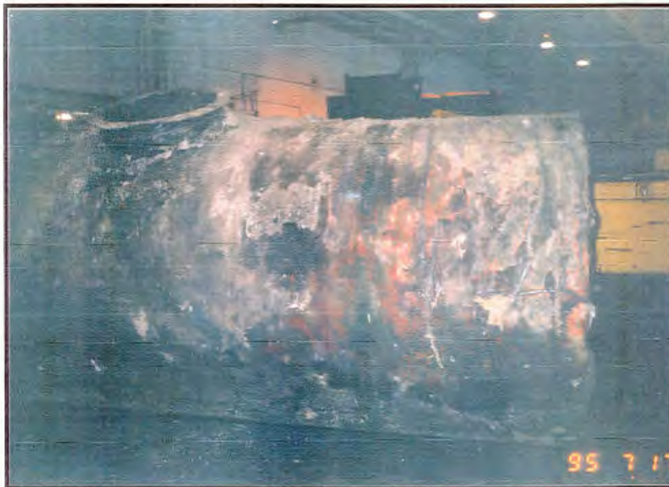
Tank 9 removed from excavation.
