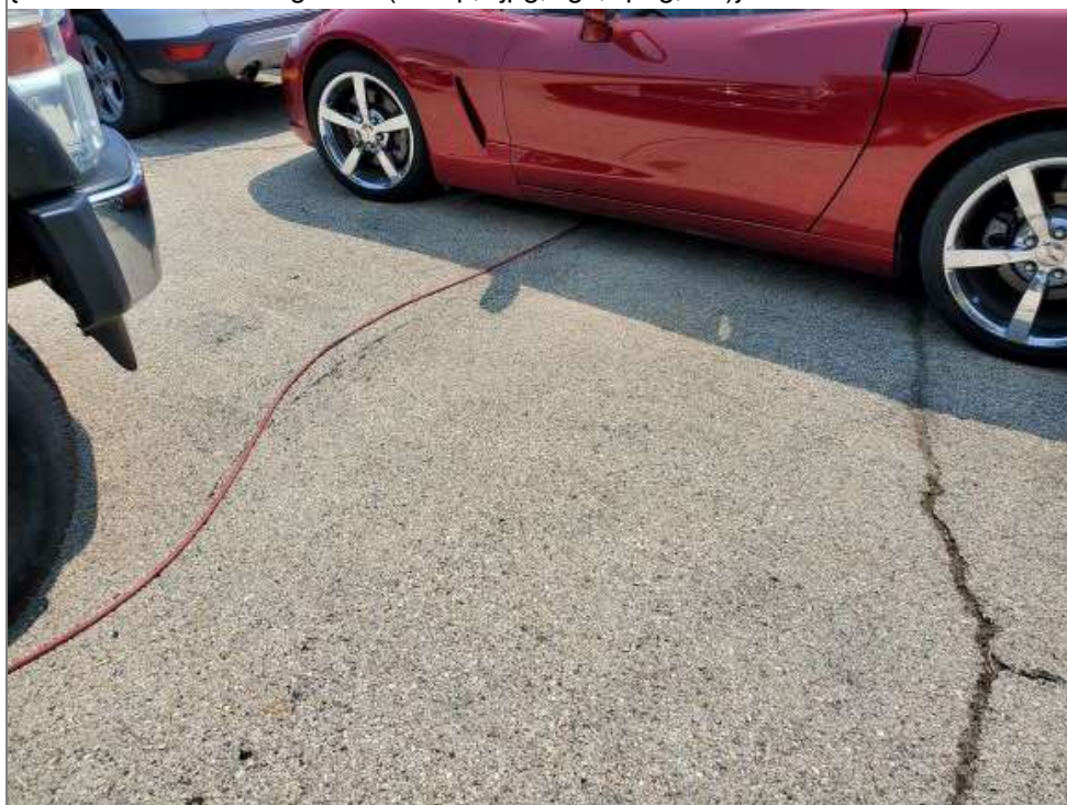
Title: Capped area, facing south from southwest corner of the building.
