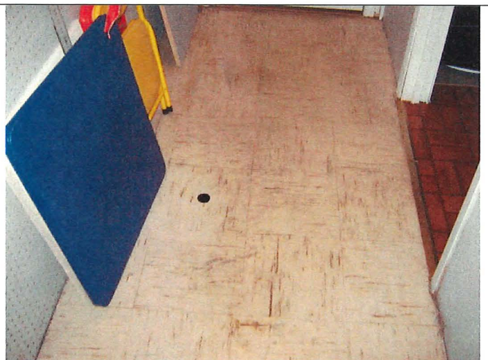
Photo 10: Flush mount cap at SSV-2.
