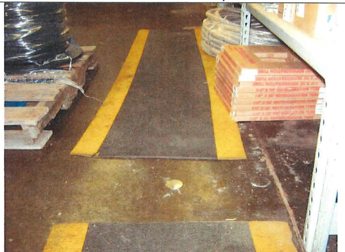
Photo 16: Flush mount cap at SSV-4.
