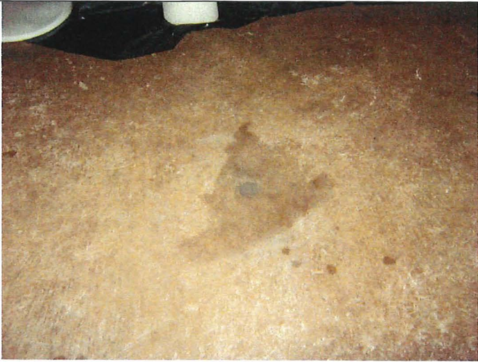
Photo 31: Vapor Pin removed and concrete patched at SSV-8.
