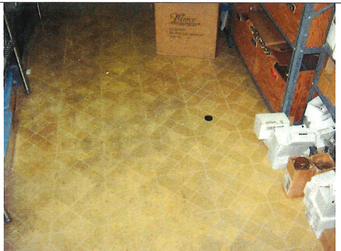
Photo 8: Flush mount cap at SSV-1.
