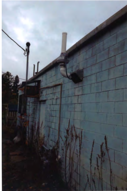
Photo 9: Fan and discharge behind Village Clippers.
