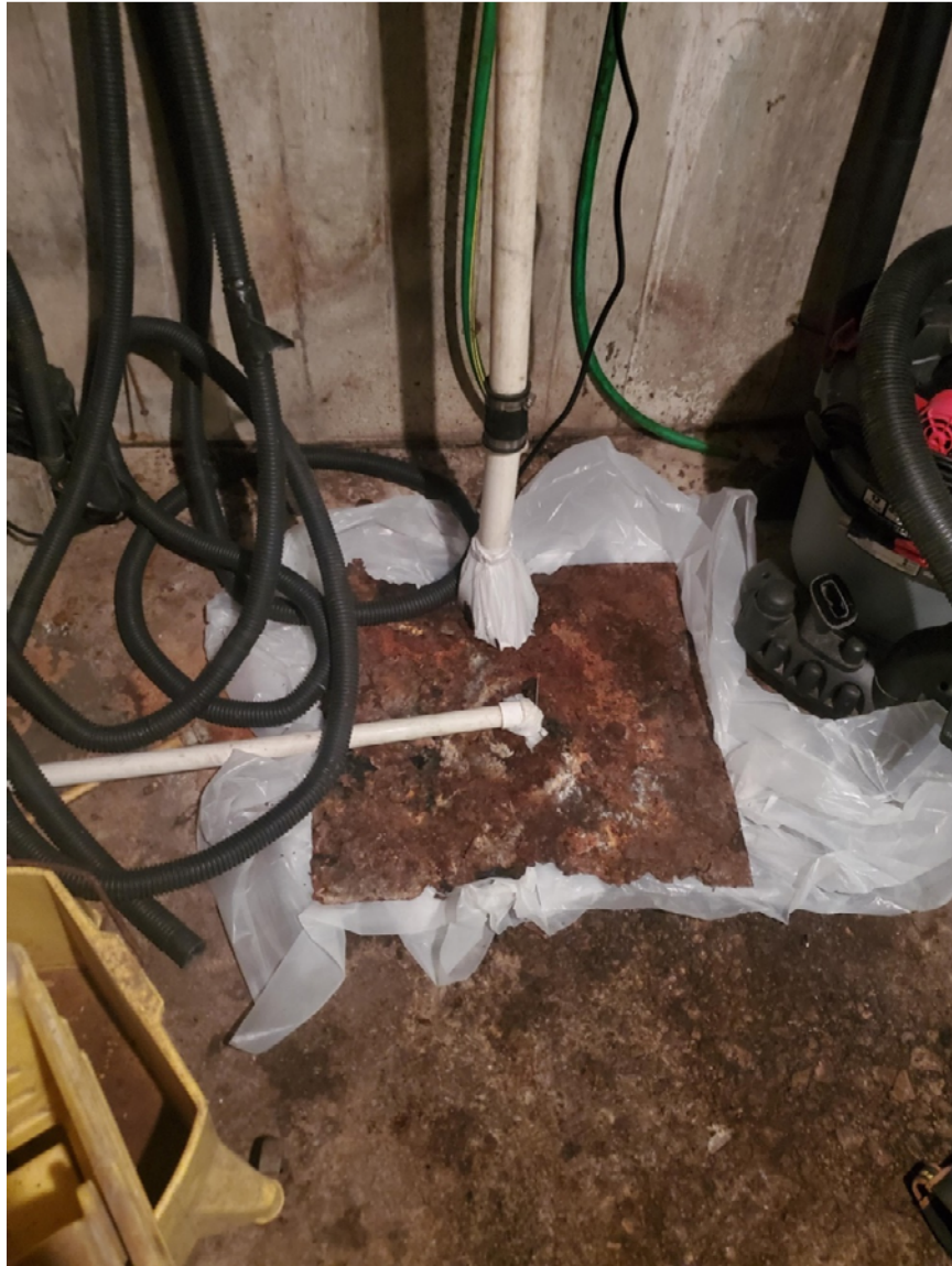
Basement sump with sealed with plastic sheeting in preparation for headspace vapor sampling.
