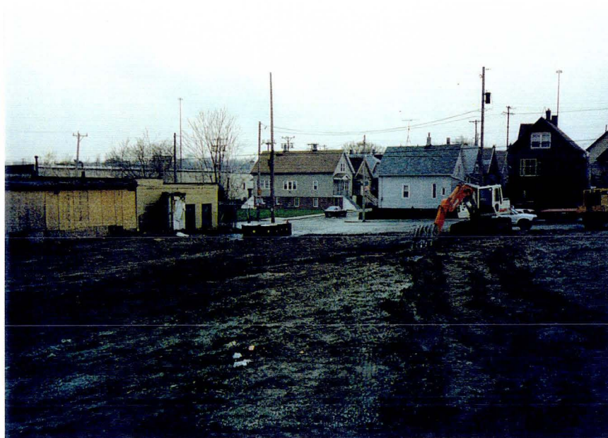
Photograph 1: Facility, looking west
