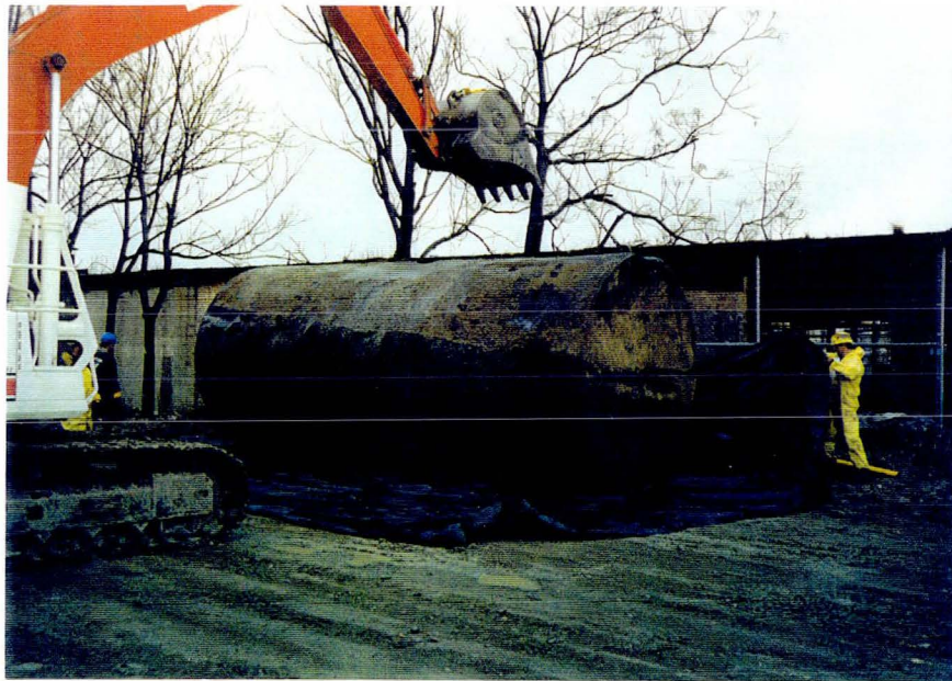
Photograph 4: Cleaned UST ready for transport
