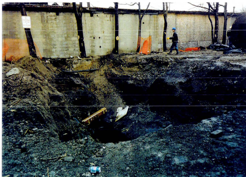
Photograph 2: Heating oil UST basin
