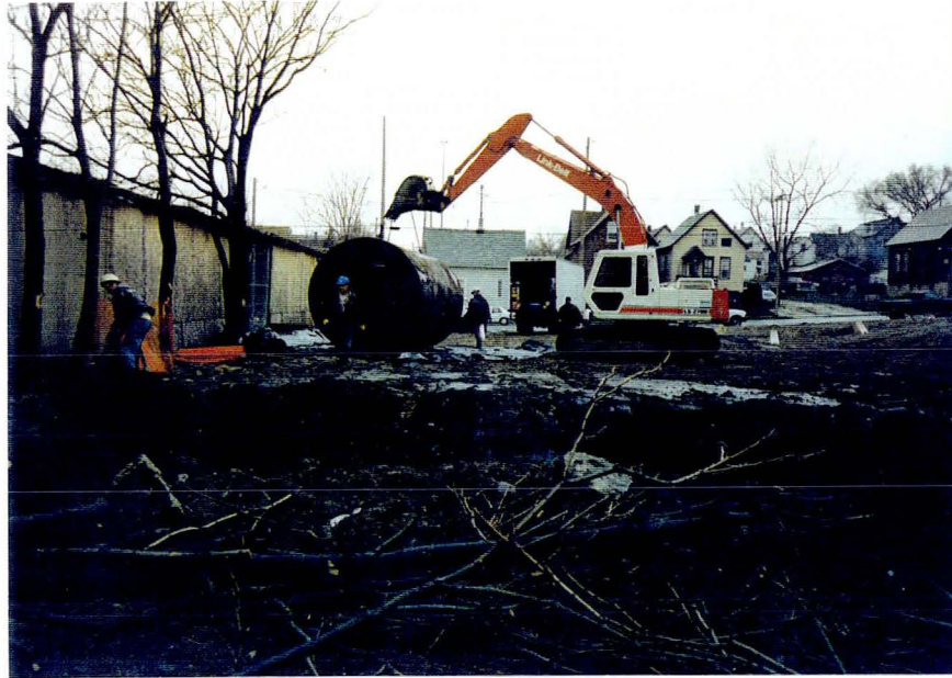
Photograph 3: Cleaning the UST
