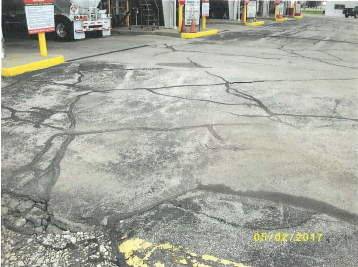
Barrier (View Southeast)
