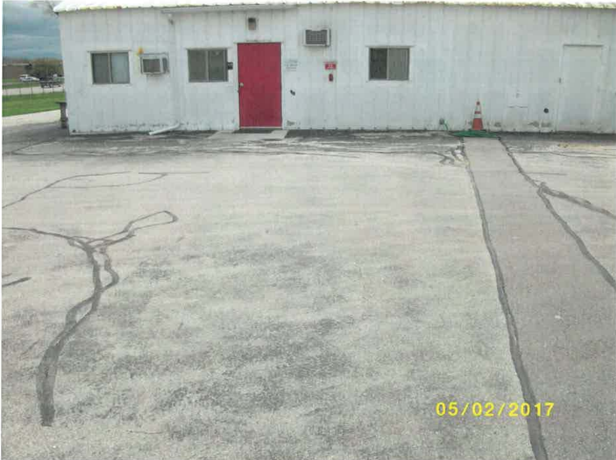
Barrier (View South)
