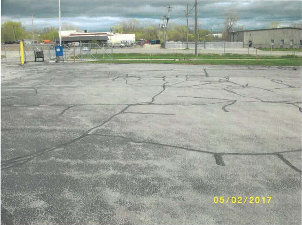
Barrier (View East)
