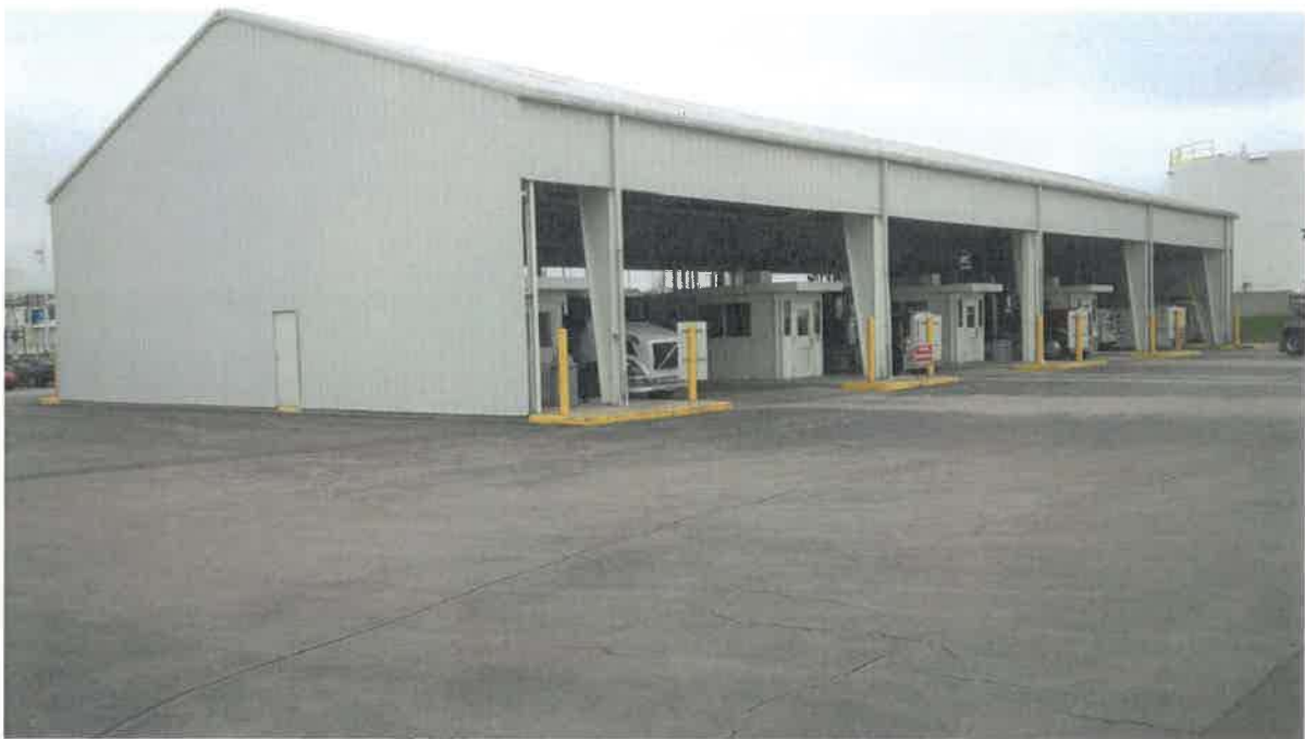
Photograph 1 – Structural Impediment (View Northwest)
