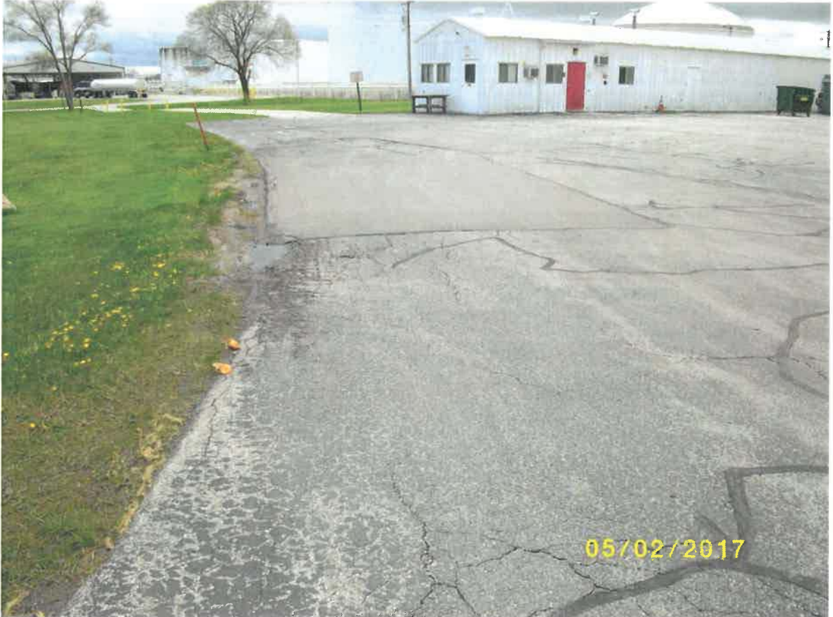
Barrier (View Southwest)
