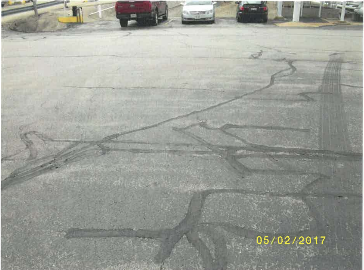
Barrier (View West)
