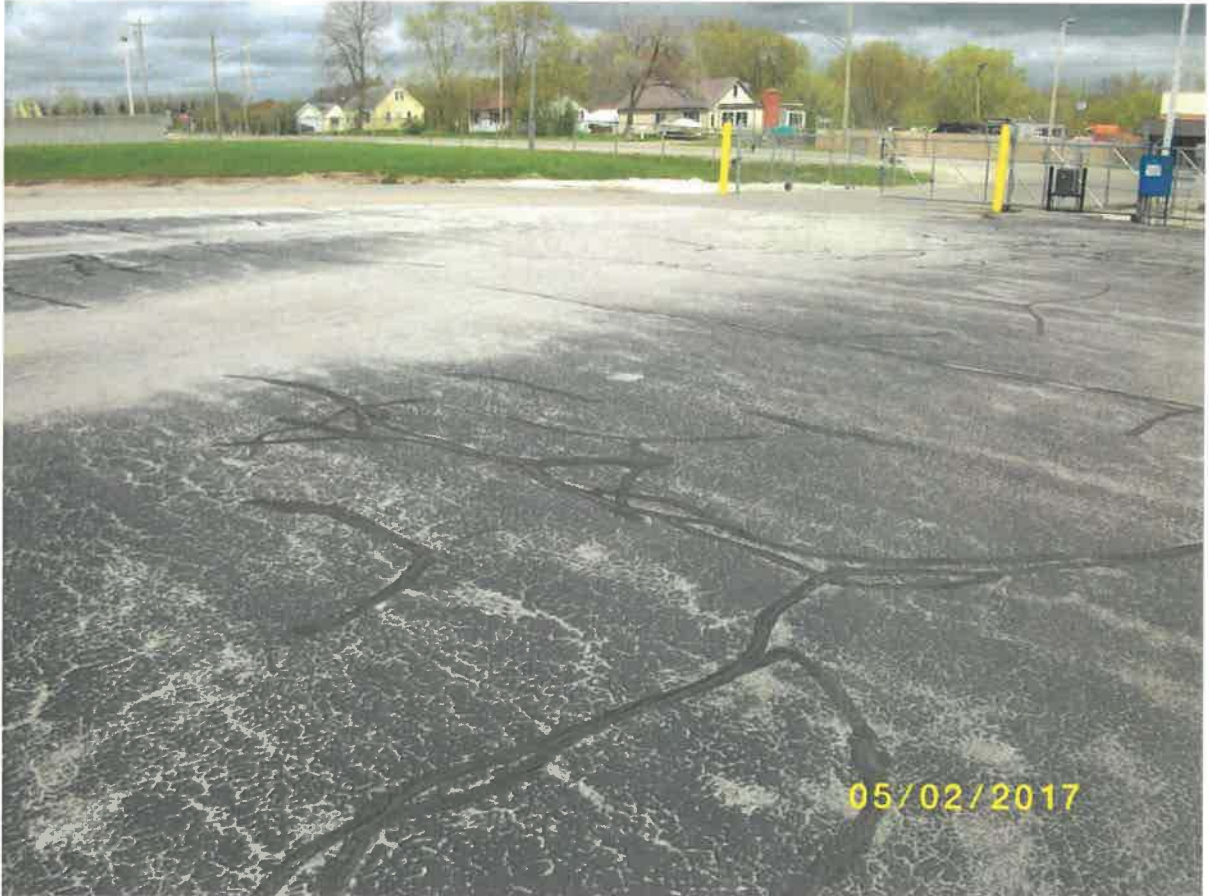
Barrier (View Northeast)
