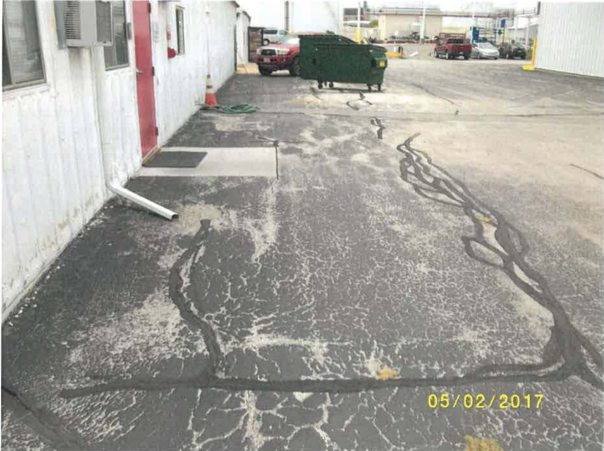
Barrier (View West)
