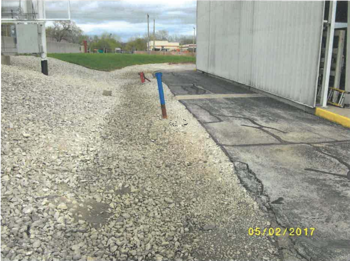
Barrier (View East)
