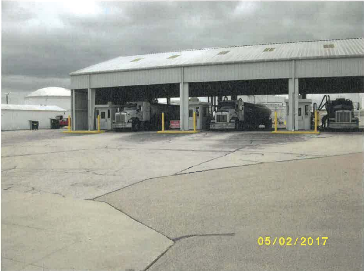
Structural Impediment (View Southwest)
