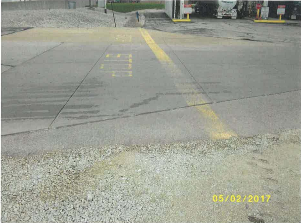
Barrier (View East)
