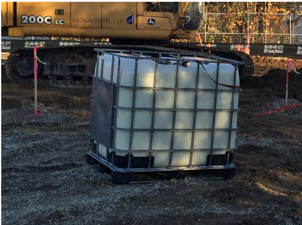
Photo 4: Typical 250-gallon tote of Anaerobic BioChem (ABC®) substrate.
