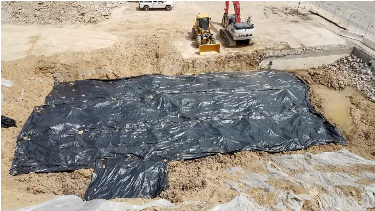
Photo 6: Geo-textile fabric placed on soil treatment area. Photograph looking east.
