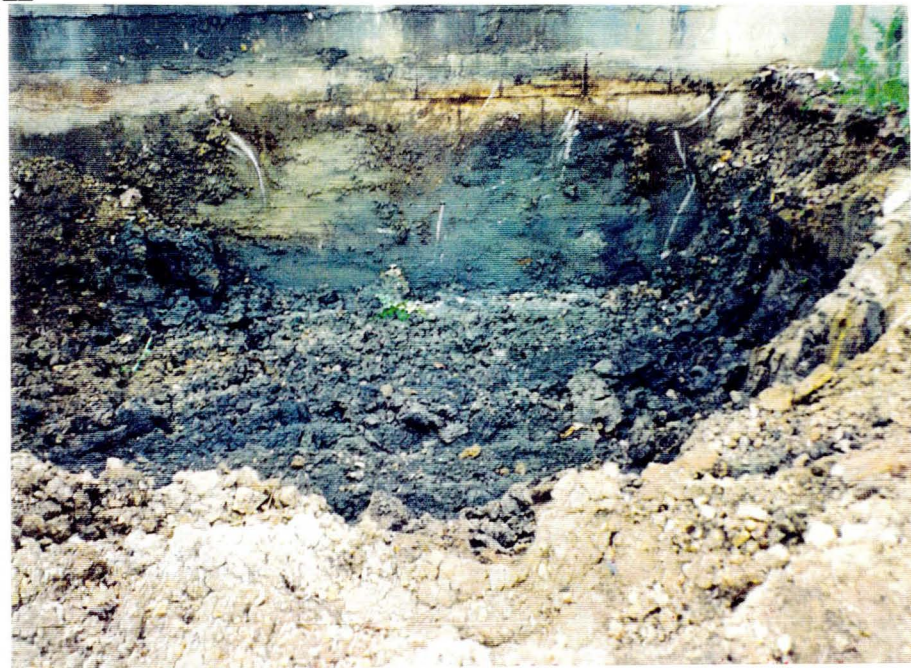
Photo #6 - Excavation area after soil removal
