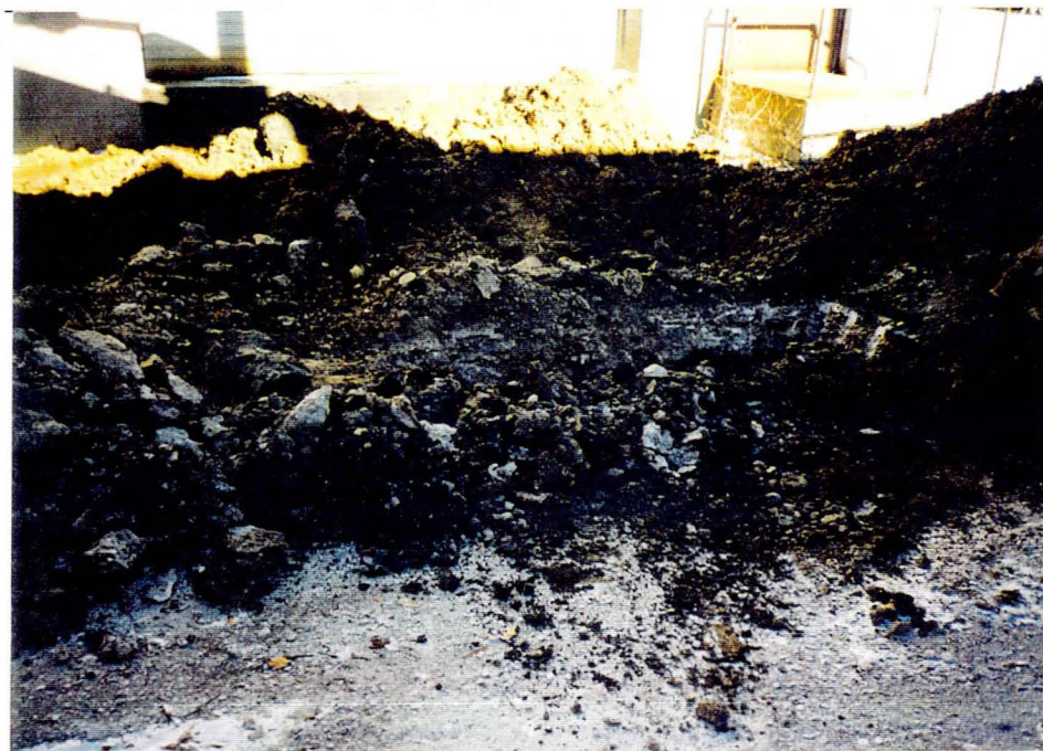
Photo #3 - Excavation area 10 ft. south of the building
