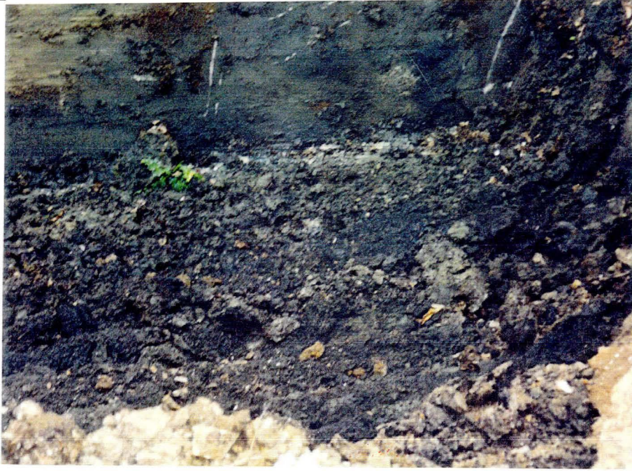
Photo #7 - Excavation area near building
