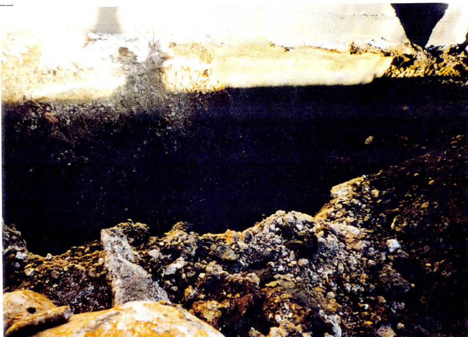
Photo #2 - Initial excavation to determine contamination
