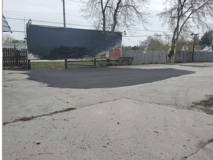
Title: Replaced pavement & surrounding existing pavement cap looking NE
