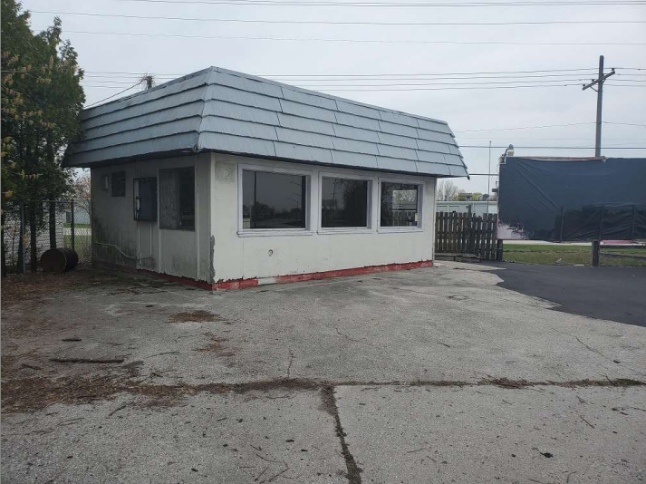
Title: Existing building foundation cap looking north.
