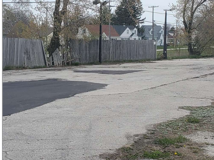
Title: Replaced paved area of former dispenser area looking northeast
