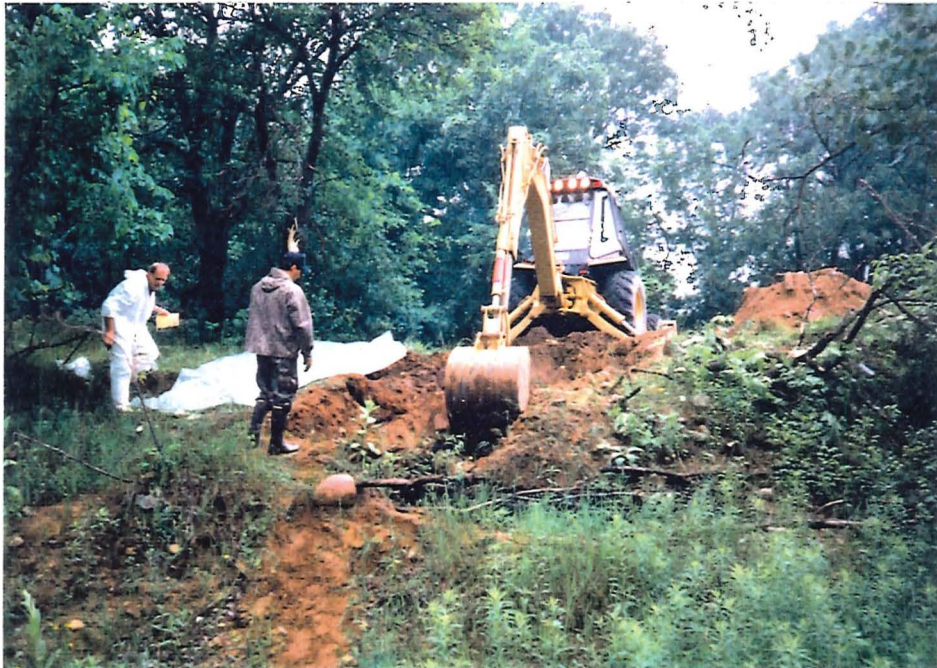
Photo 3: Test Pit and Staging Area
