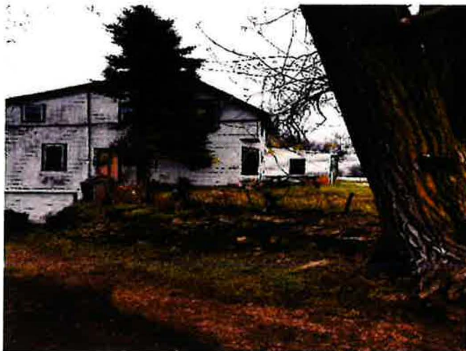
PHOTOGRAPH OF LARGE TREE, HOUSE, AND RETAINING WALL PRESENT WITHIN/NEAR THE LIMITS OF THE PLANNED EXCAVATION
