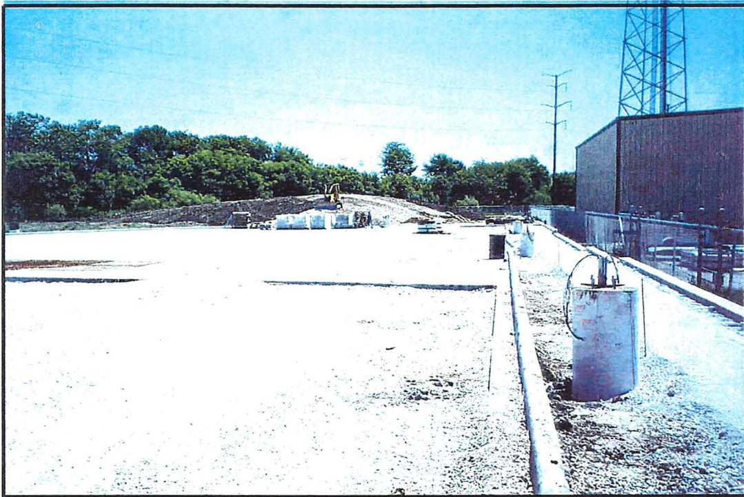
Excess material berm construction.
