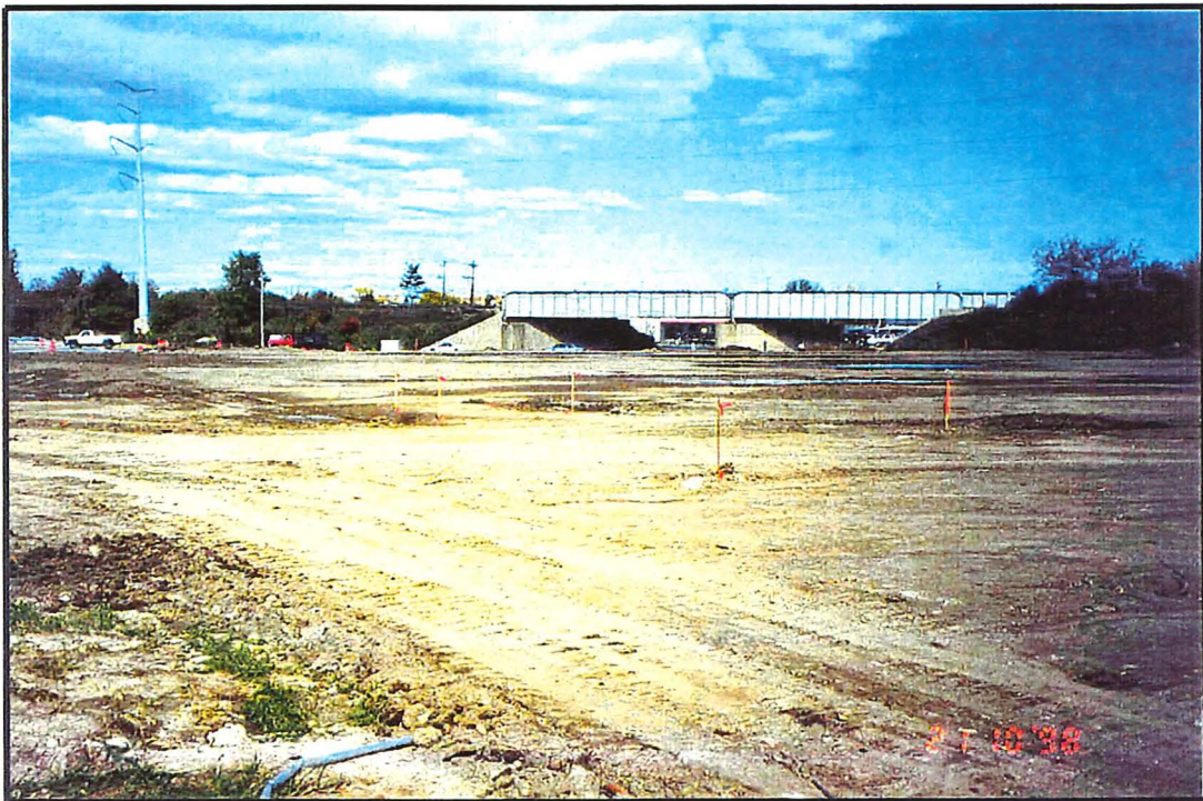
Completed grading of building footprint.
