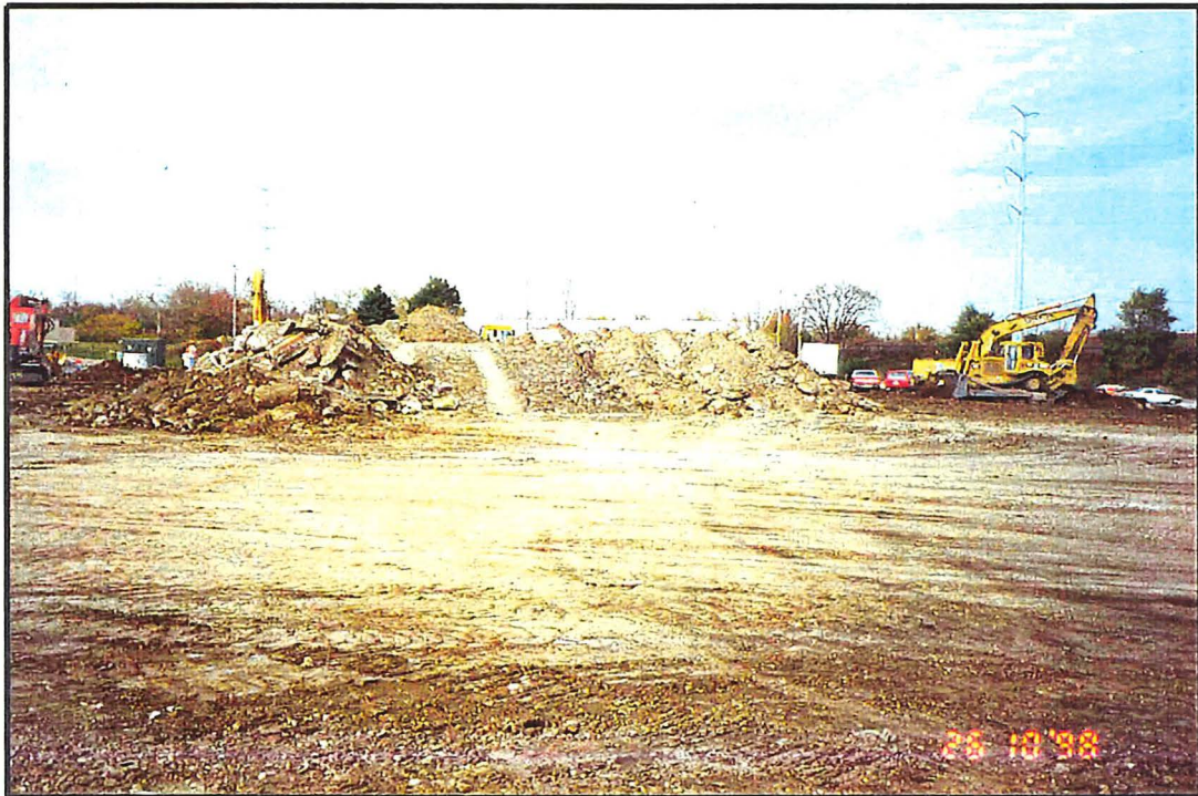
Excess material stockpile.
