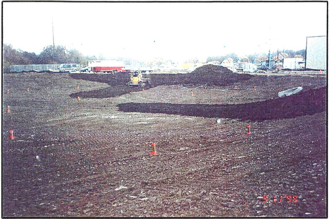
Placement of clean fill.
