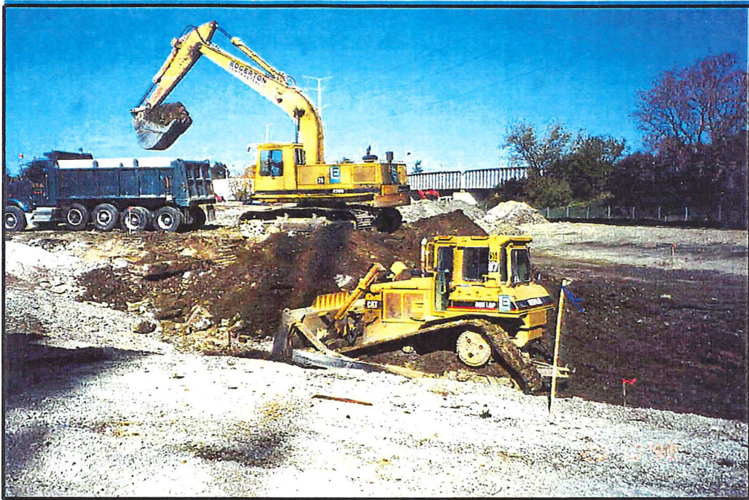
Excavation for detention pond.
