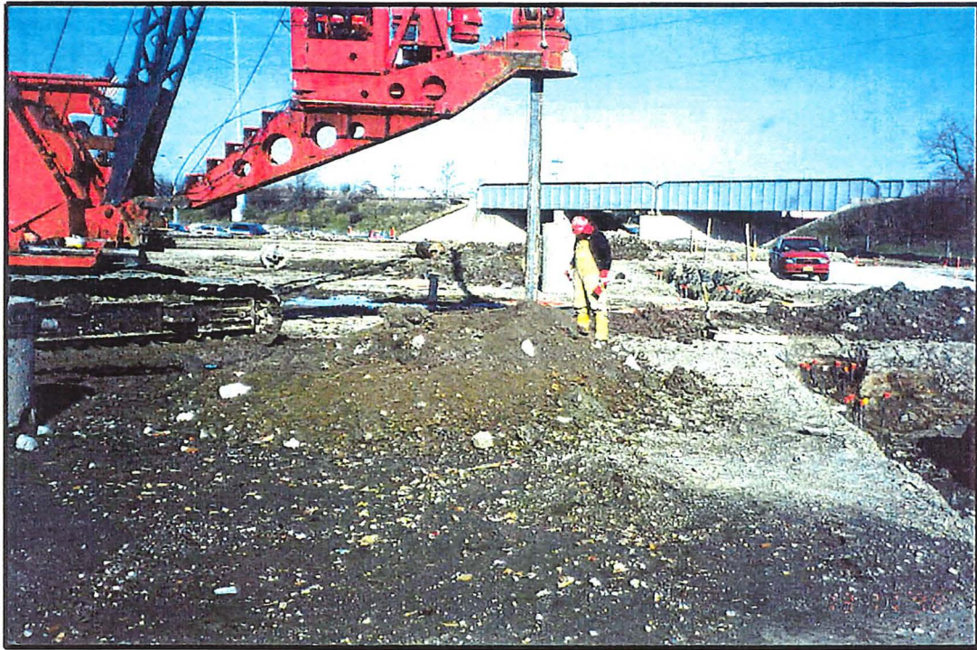
Caisson drilling.
