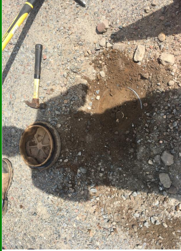
MW4 - flushmount lid detached from skirt and vault filled with debris
