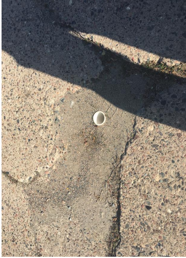
MW2 - Before and After. MW2 will need a new flushmount well vault installed
