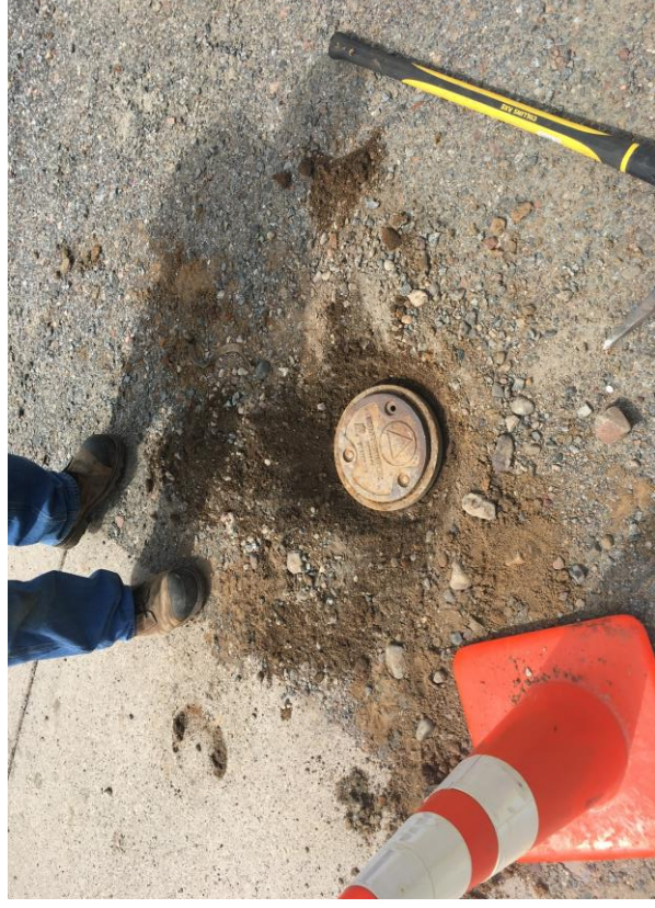
MW4 - flushmount lid detached from skirt and vault filled with debris
