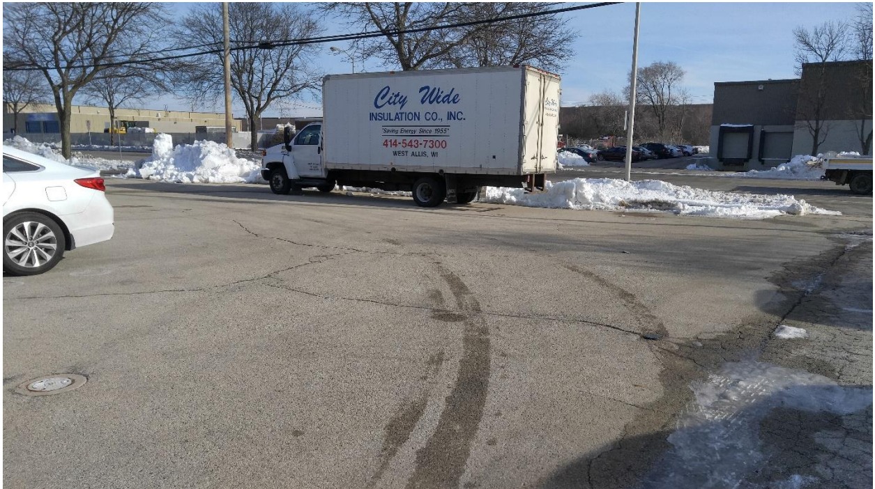
EASTERN PORTION OF THE IMPERMEABLE CAP LOOKING NORTHEAST
