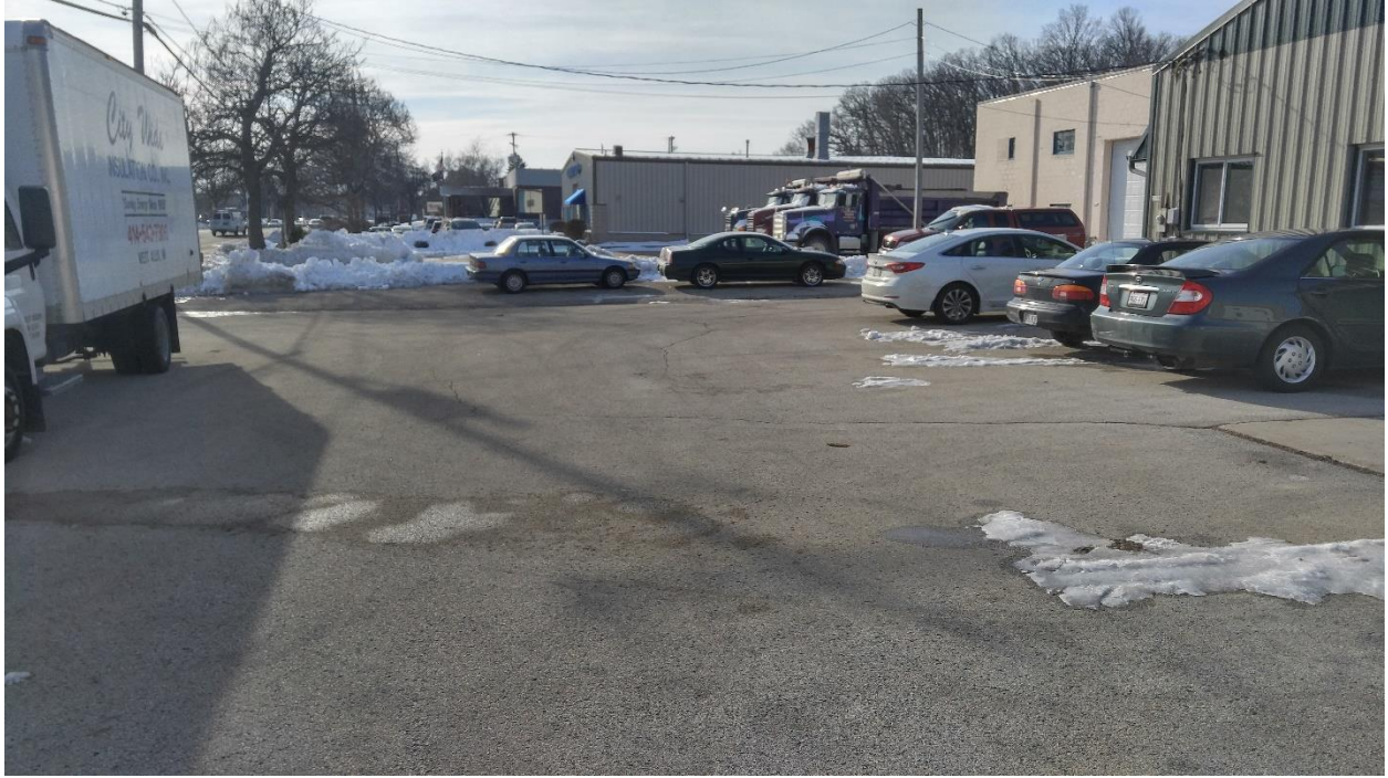
NORTHERN PORTION OF THE IMPERMEABLE CAP LOOKING SOUTH
