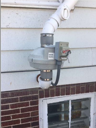
Title: Fan on north side of house - red switch in "on" position
