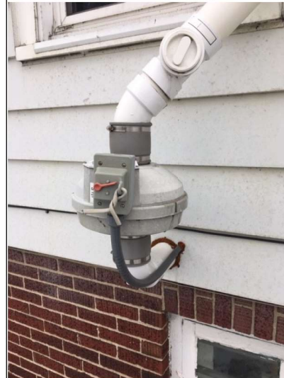
Title: Fan on north side of house - red switch in "on" position
