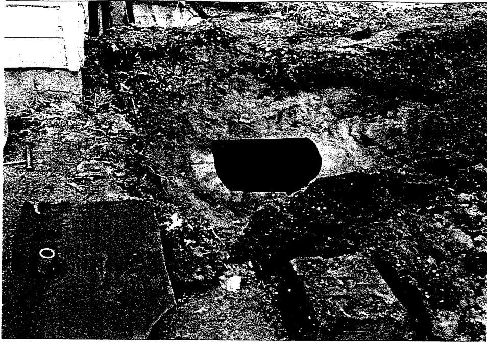
Waubeka Mill UST uncovered with top cut off.
