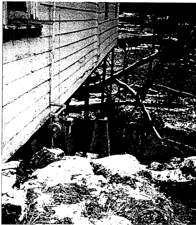
Looking North along east side of mill. The Milwaukee River is visible in the background.
