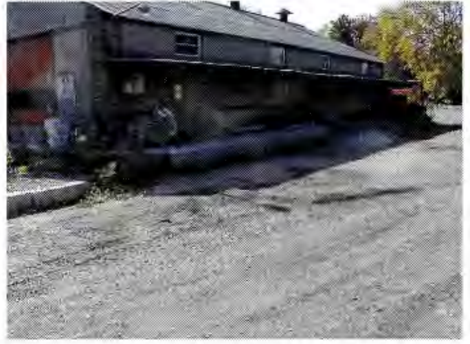
Petroleum stain outside bldg 2
