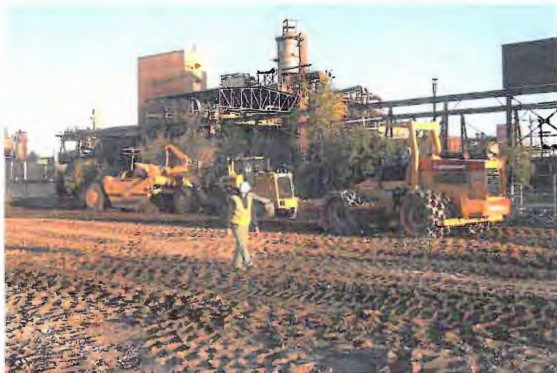
PHOTOGRAPH 20: Site Grading and Earthwork: Site backfill and compaction.
