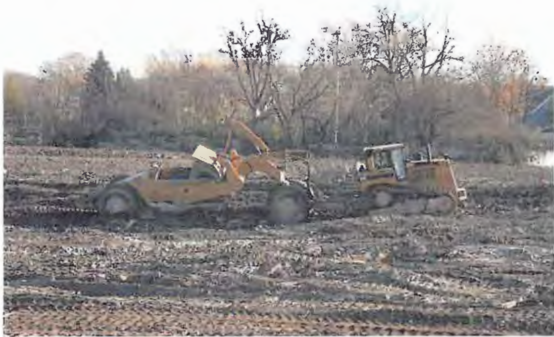
PHOTOGRAPH 23: Site Grading and Earthwork: Wet detention pond excavation.
