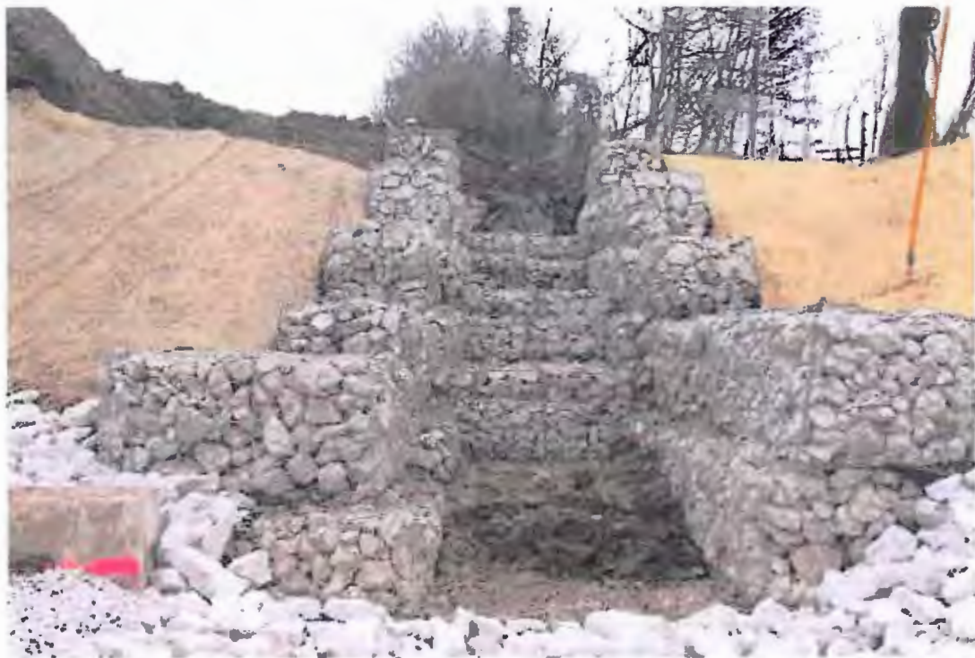
PHOTOGRAPH 28: Gabion-Lined Channel: Gabion-lined channel installation and restoration, photo taken looking west.
