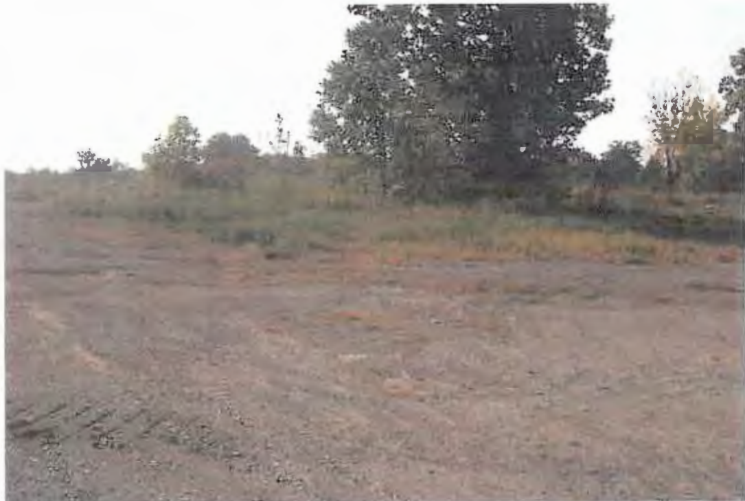
PHOTOGRAPH 2: Pre Site Grading and Earthwork: Burnham entrance looking southeast.
