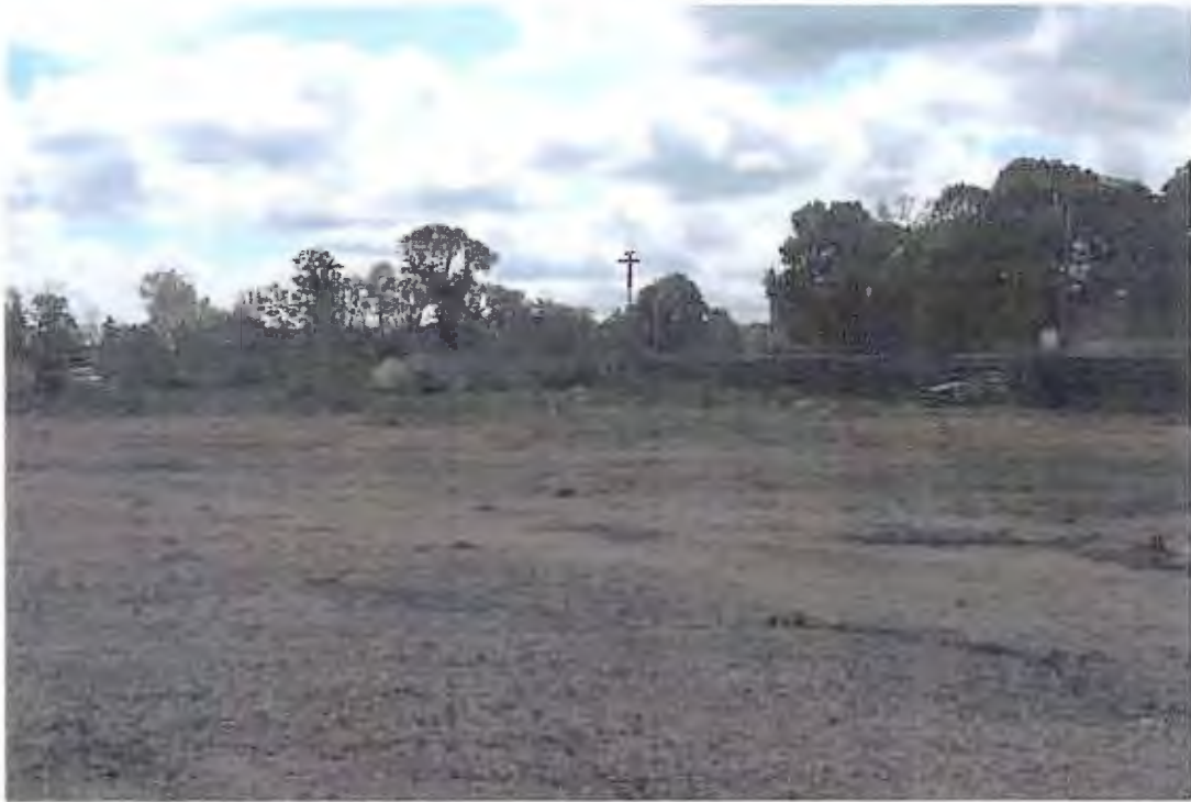
PHOTOGRAPH 7: Clearing and Grubbing: Stump grinding along western Site perimeter.
