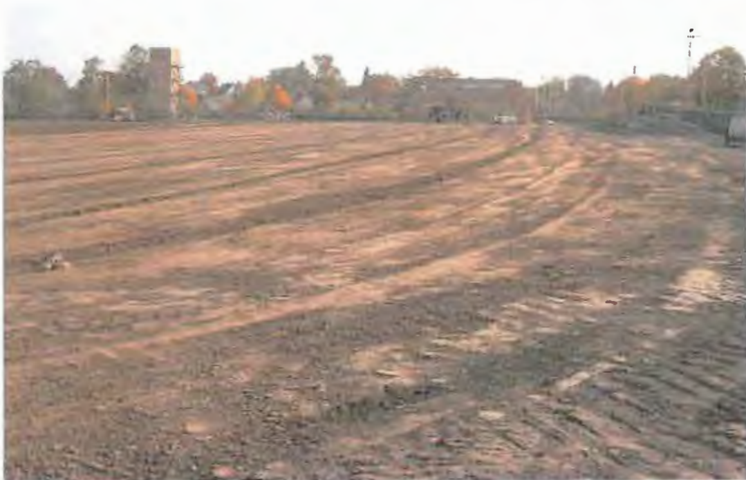
PHOTOGRAPH 21: Site Grading and Earthwork: Site backfill and compaction.
