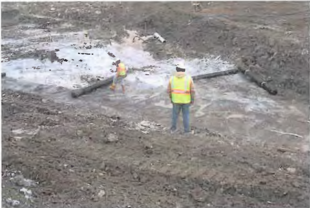
PHOTOGRAPH 34: Wet Detention Pond Installation: Bridge lift construction, Tensor BX 1200 Geogrid installation.
