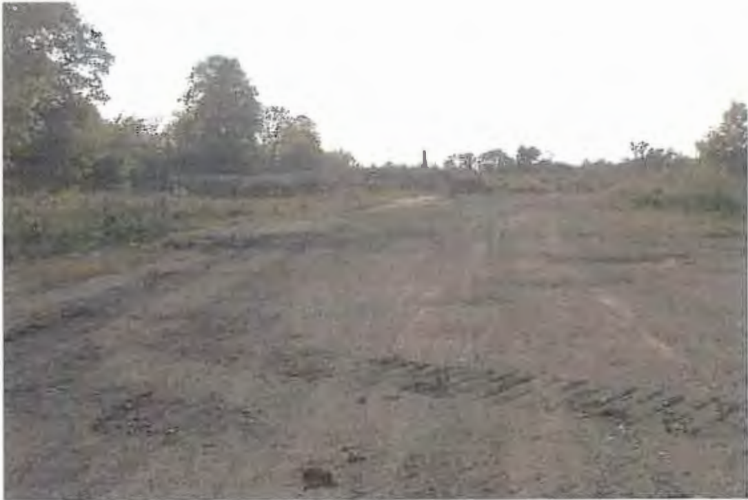
PHOTOGRAPH 1: Pre Site Grading and Earthwork: Burnham entrance looking east.
