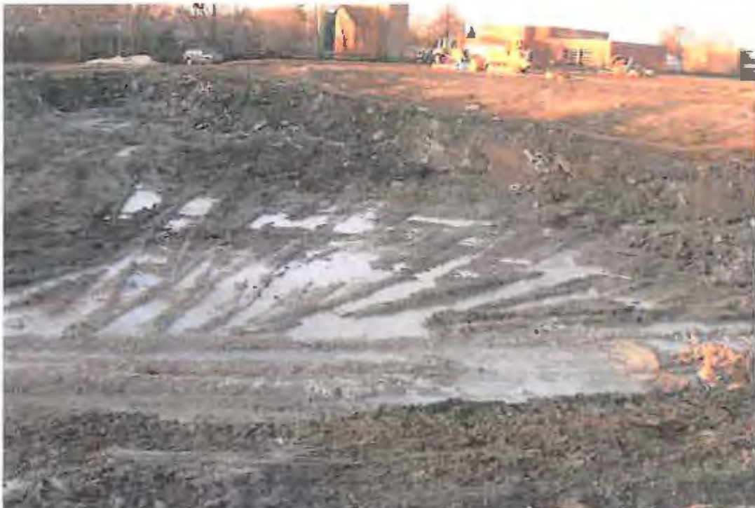
PHOTOGRAPH 26: Site Grading and Earthwork: Wet detention pond excavation, original excavation extent.
