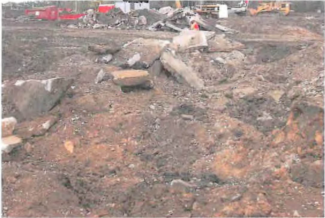
PHOTOGRAPH 13: Surface Debris: Foundation and concrete slab removal per specifications.
