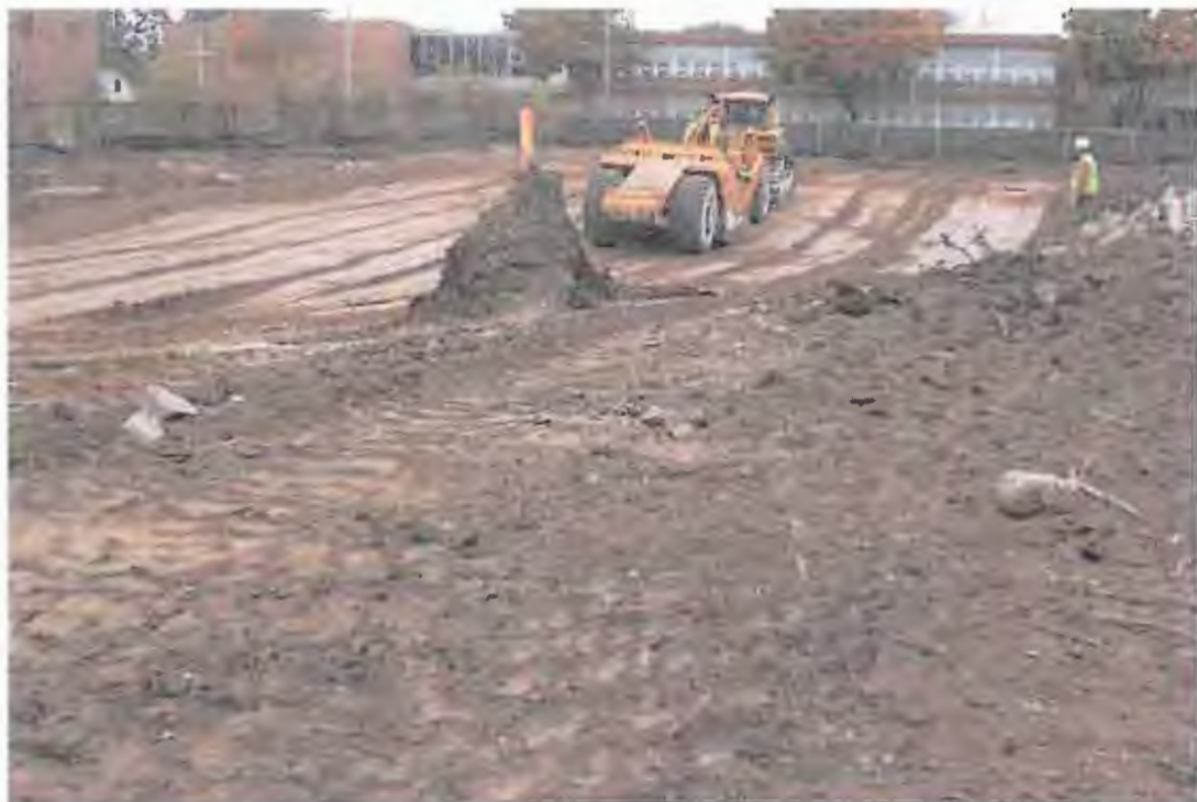
PHOTOGRAPH 19: Site Grading and Earthwork: Borrow pit excavation.
