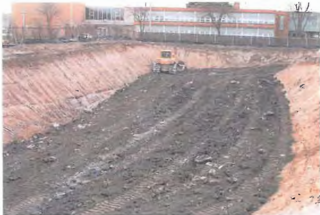
PHOTOGRAPH 24: Site Grading and Earthwork: Borrow pit backfill.
