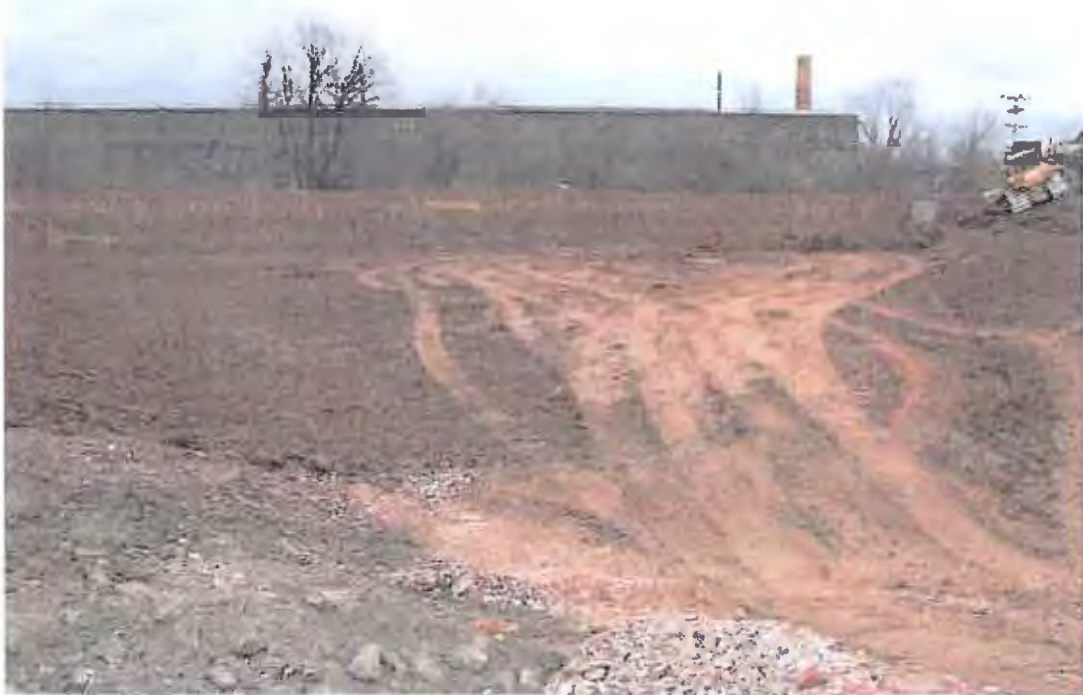
PHOTOGRAPH 36: Wet Detention Pond Installation: Clay liner installation, photograph taken looking north.
