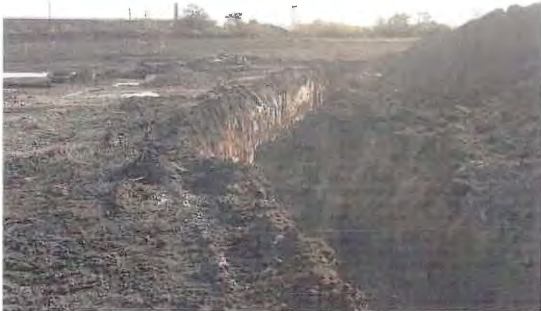
PHOTOGRAPH 15: Sprinkler Vault: Discharge piping removed per specifications.
