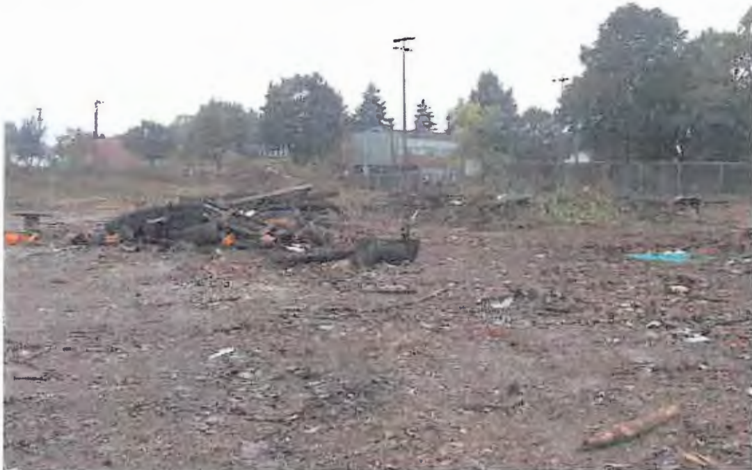
PHOTOGRAPH 11: Surface Debris: Surface debris removal per specifications.
