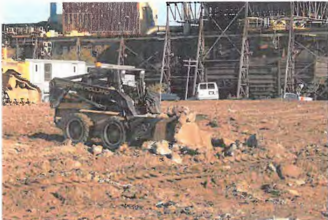
PHOTOGRAPH 18: Site Grading and Earthwork: Backfill screening/raking.
