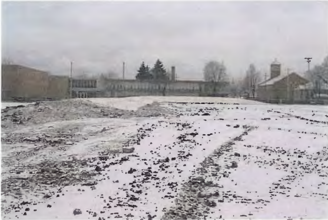
PHOTOGRAPH 41: Site Restoration: South and southwestern berm, photograph taken looking west.
