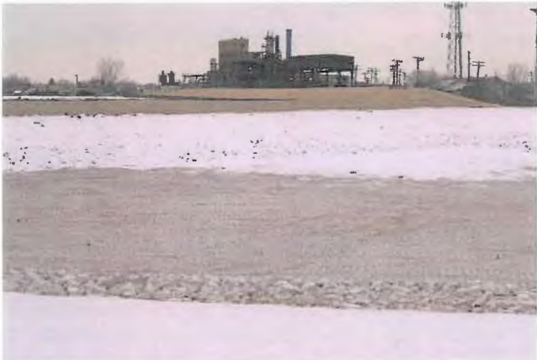
PHOTOGRAPH 42: Site Restoration: Wet detention pond and northern berm, photograph taken looking northwest.
