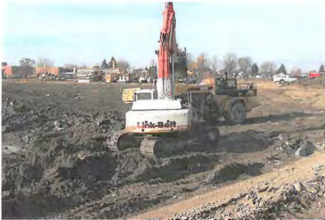
PHOTOGRAPH 25: Site Grading and Earthwork: Wet detention pond excavation.
