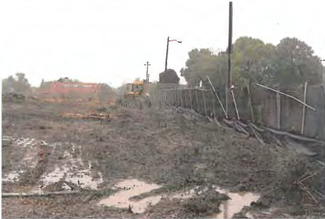
PHOTOGRAPH 9: Stormwater Controls: Western perimeter silt fence.
