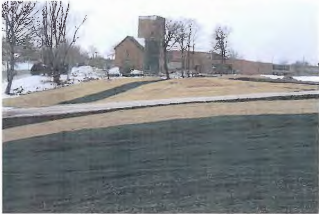
PHOTOGRAPH 39: Southeast Ditch: Ditch installation and restoration complete, photograph taken looking south.
