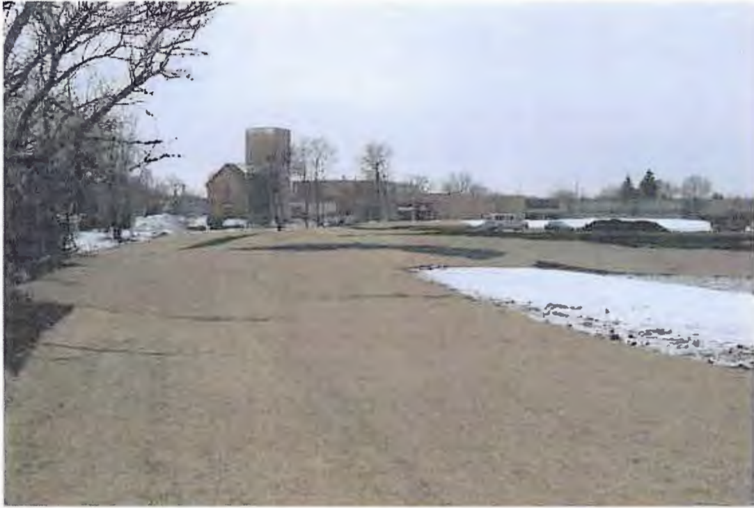
PHOTOGRAPH 43: Site Restoration: Wet detention pond, spillway, and southeast ditch, photograph taken looking south.
