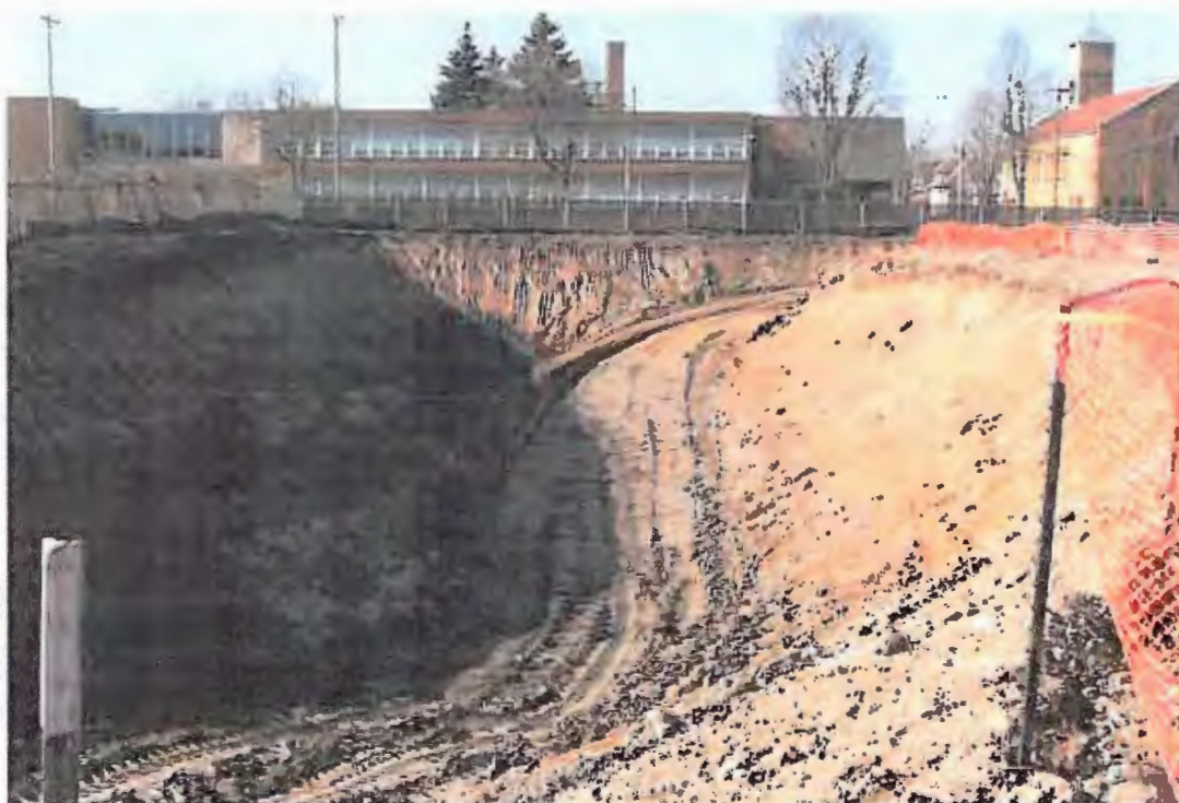
PHOTOGRAPH 22: Site Grading and Earthwork: Final extent of borrow pit excavation.
