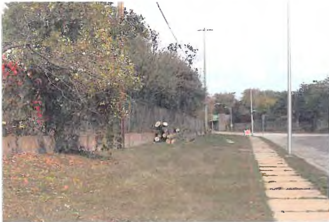
PHOTOGRAPH 8: Clearing and Grubbing: Tree removal along West Becher Place.
