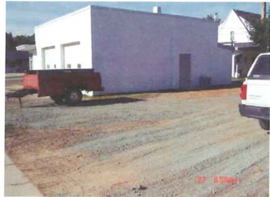
Photo 2 North Gravel Cover
