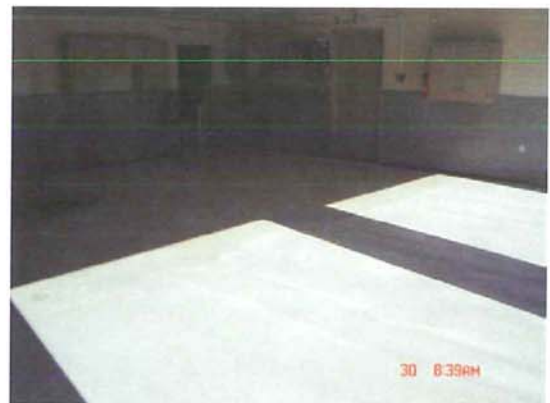
Photo 6 Interior of Garage
