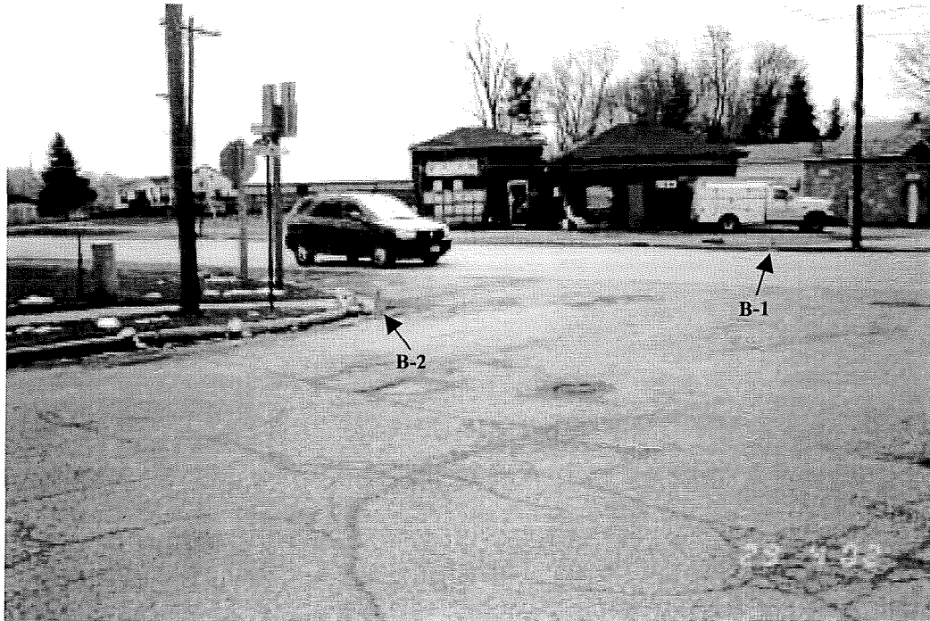
View southwest of A-Z Sales and Service at the corner of CTH A and Main Street. The orange cones indicate the locations of Soil Borings B-1 (right cone) and B-2 (left cone).
