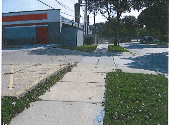
Looking E along S side of building.
