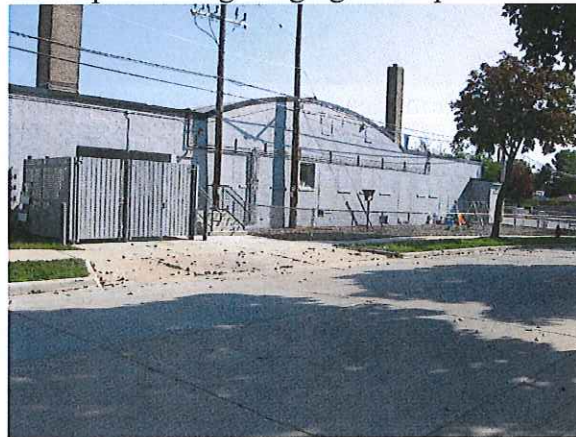
E portion of S side of building.
