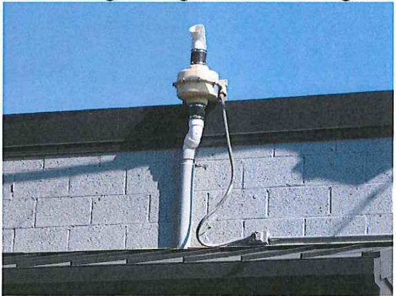
Vent pipe and fan assembly; close-up of same.
