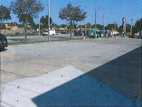
Looking NW across excavation area.
