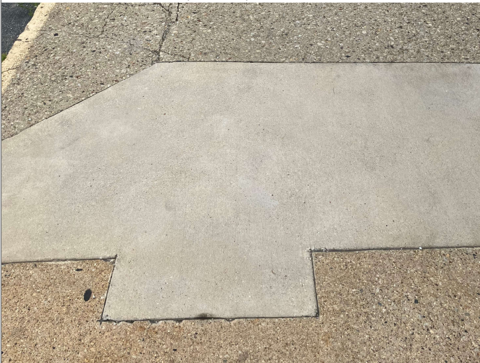
Title: Previously repaired section of the cover in fine condition.
