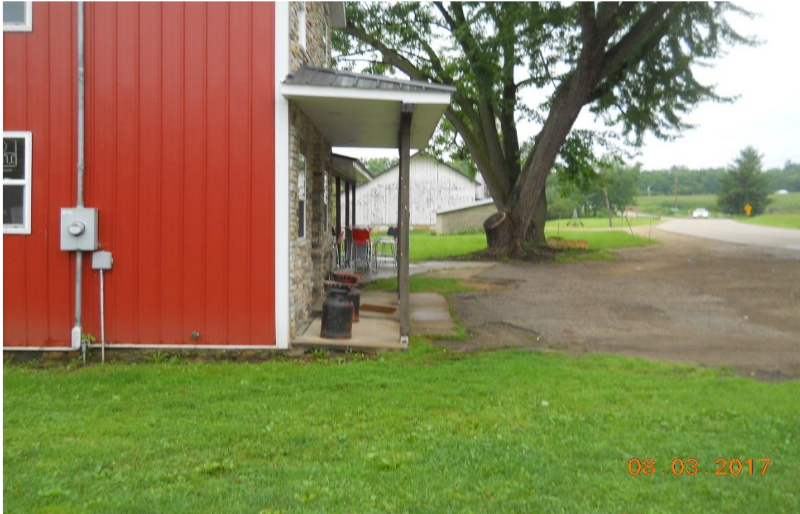
Photo #7: Looking south at the asphalt parking lot on the western side of the building (post-renovation).
