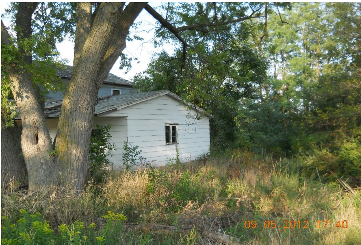
Photo #2: Looking northeast at the on-site building (pre-renovation).
