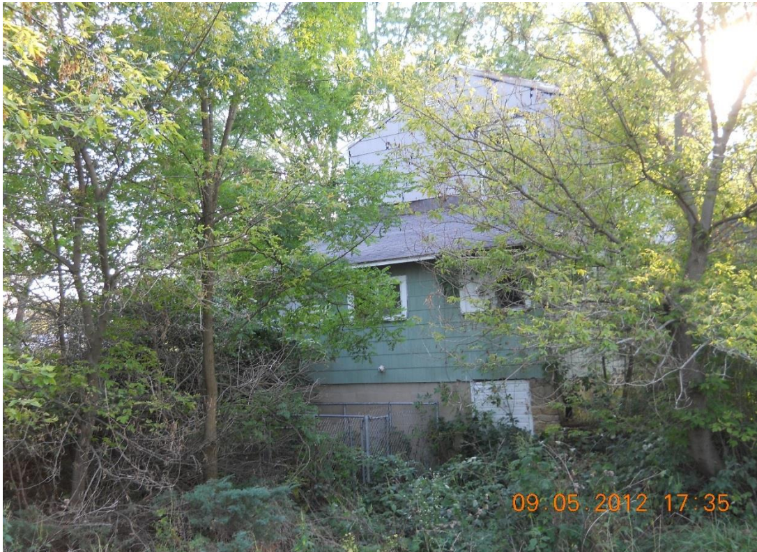
Photo #1: Looking west at the on-site building (pre-renovation).
