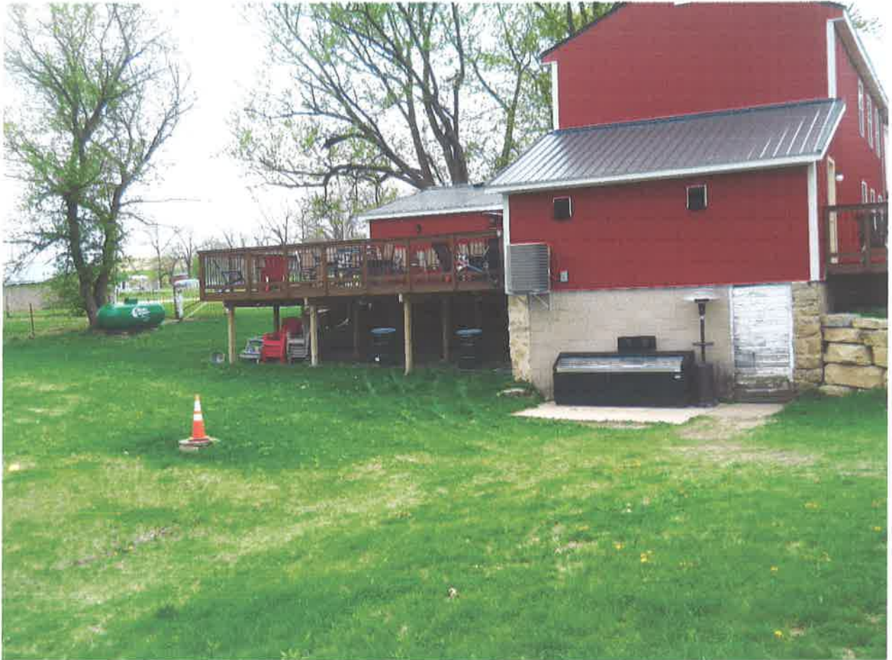
Photo #2: On site building looking southwest (picture taken: 4/25/2017).
