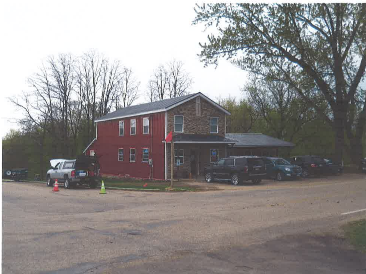
Photo #1: On site building looking southeast (picture taken: 4/25/2017).
