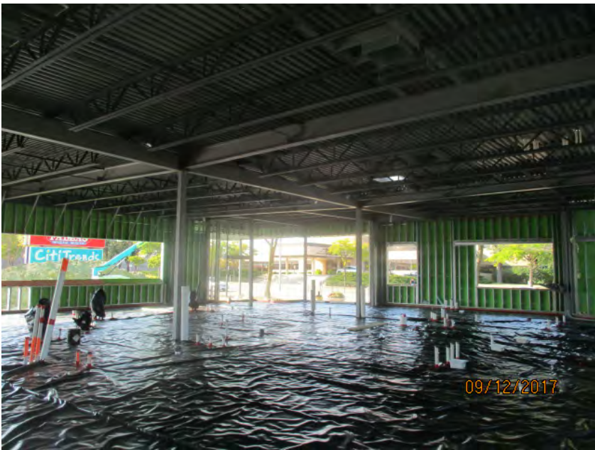
View of the 40-mil PVC liner installation.
