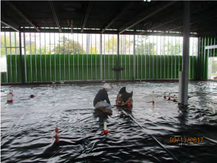
View of the 40-mil PVC liner installation showing pipe boot installation.
