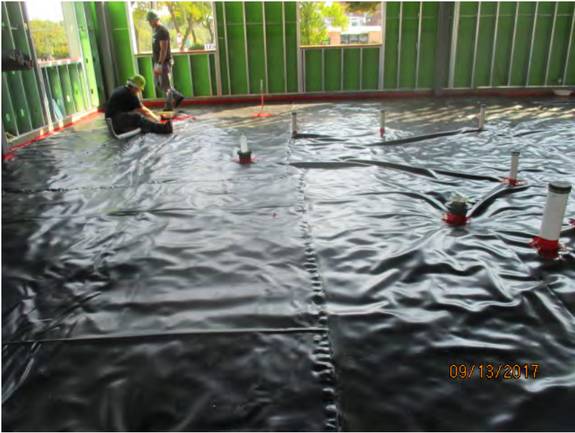
View of the 40-mil PVC liner installation showing seaming activities using solvent weld compound.
