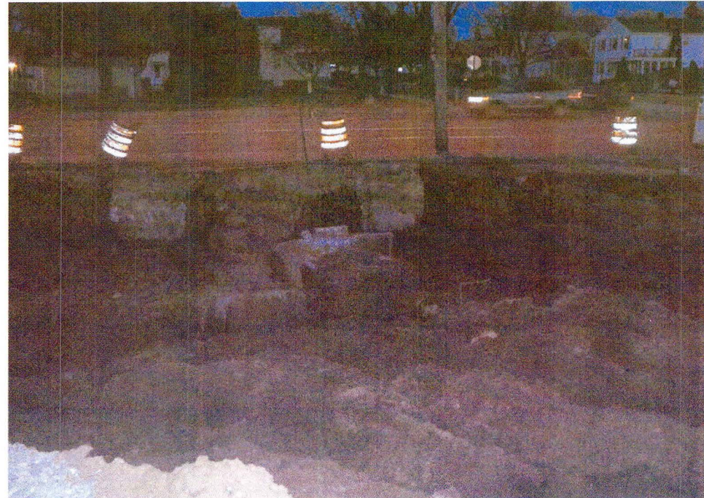
View of excavation looking north
