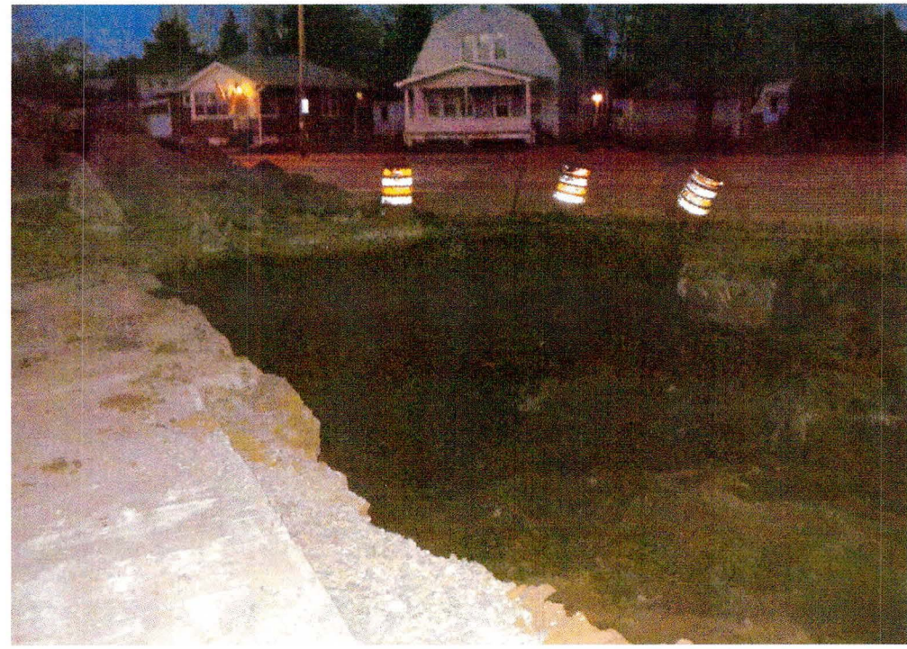
View of excavation looking north west
