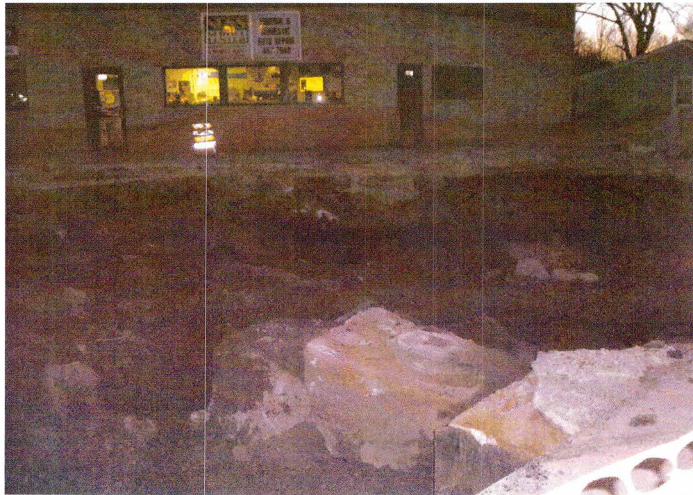
View of excavation looking south west
