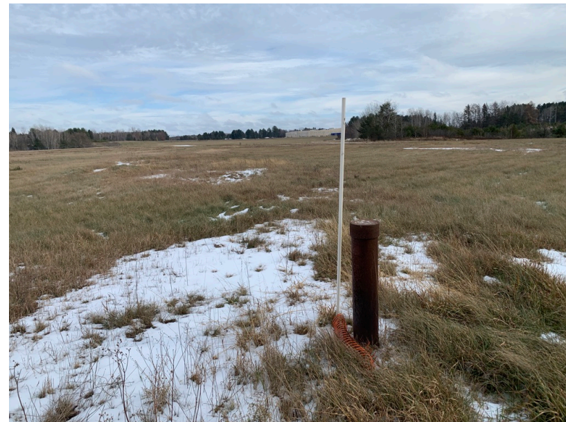
Interior Well at closed Rhineland Landfill
